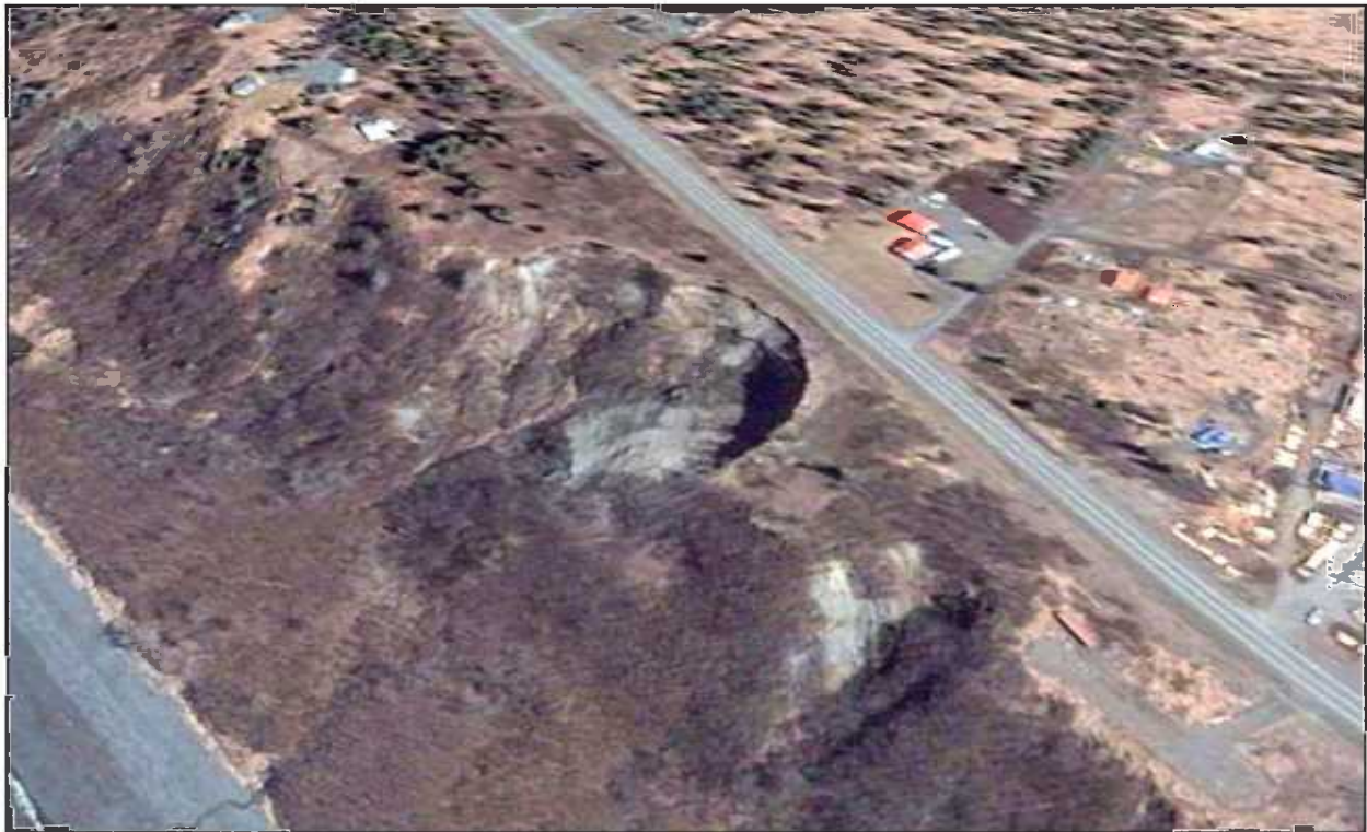
As seen in this aerial image, the eroding edge of the bluff is now only 30 feet away from the Sterling Highway at a section just north of Anchor Point.
