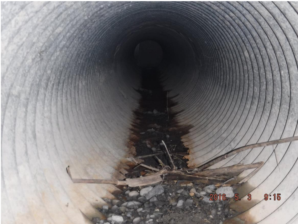
E. Bunnell Avenue – at inlet of 18-inch lead southwest of SD 246
