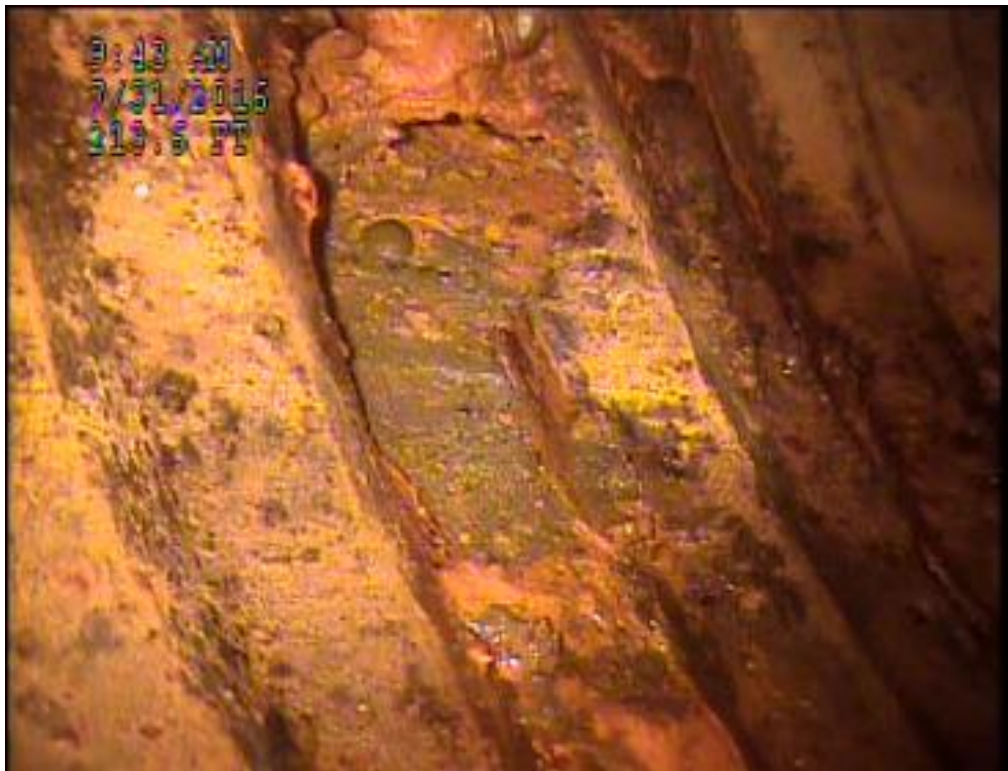
E. Bunnell Avenue – hole in 36-inch CMP
