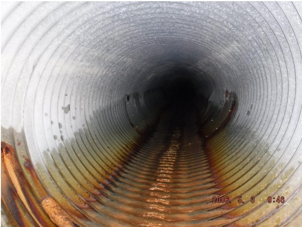
E. Bunnell Avenue – downstream 36-inch CMP at SD 244
