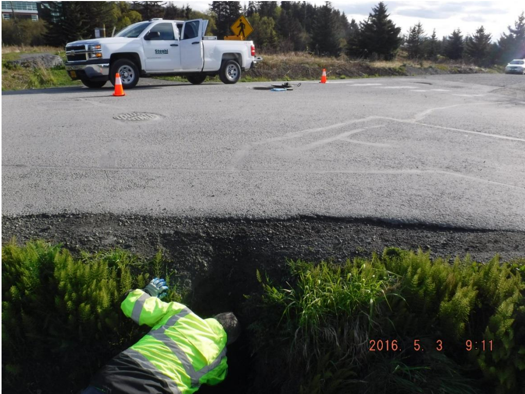
Looking northeast at 18-inch inlet to SD 246
