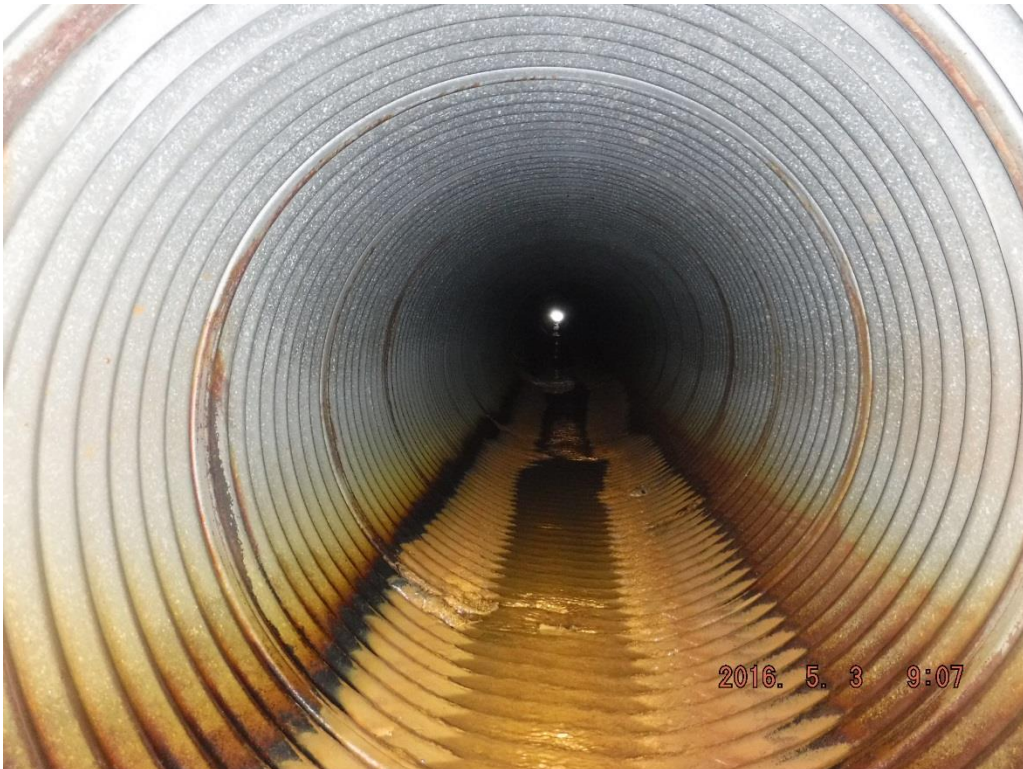
E. Bunnell Avenue – downstream 36-inch pipe at SD 246
