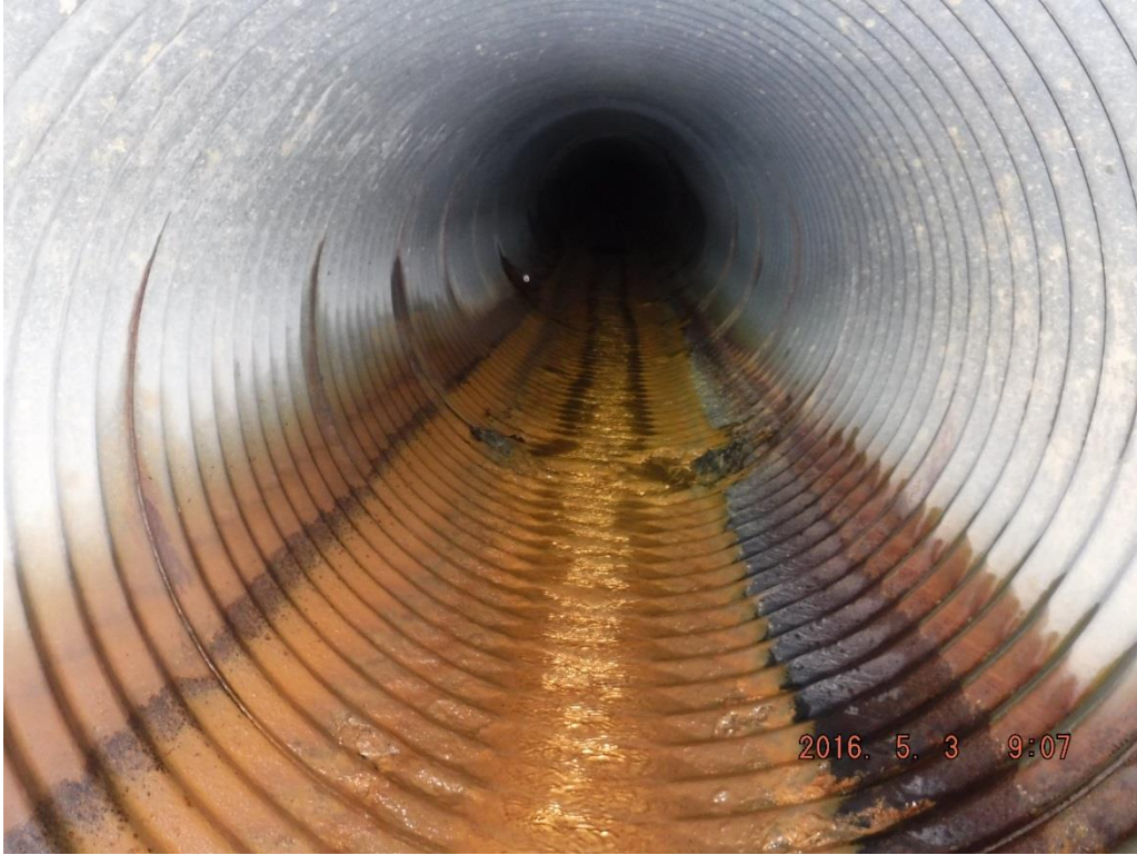
E. Bunnell Avenue – upstream 36-inch pipe at SD 246
