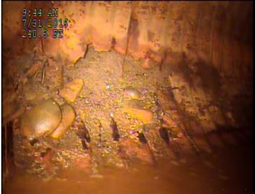
E. Bunnell Avenue – hole in 36-inch CMP
