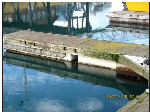
Exposed flotation on a damaged float.
