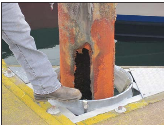
Hole in damaged piling that needs replacing
