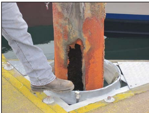
Hole in damaged piling that needs replacing
