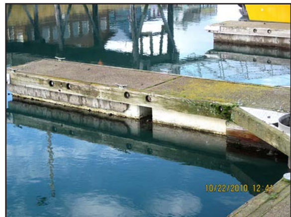
Exposed flotation on a damaged float.
