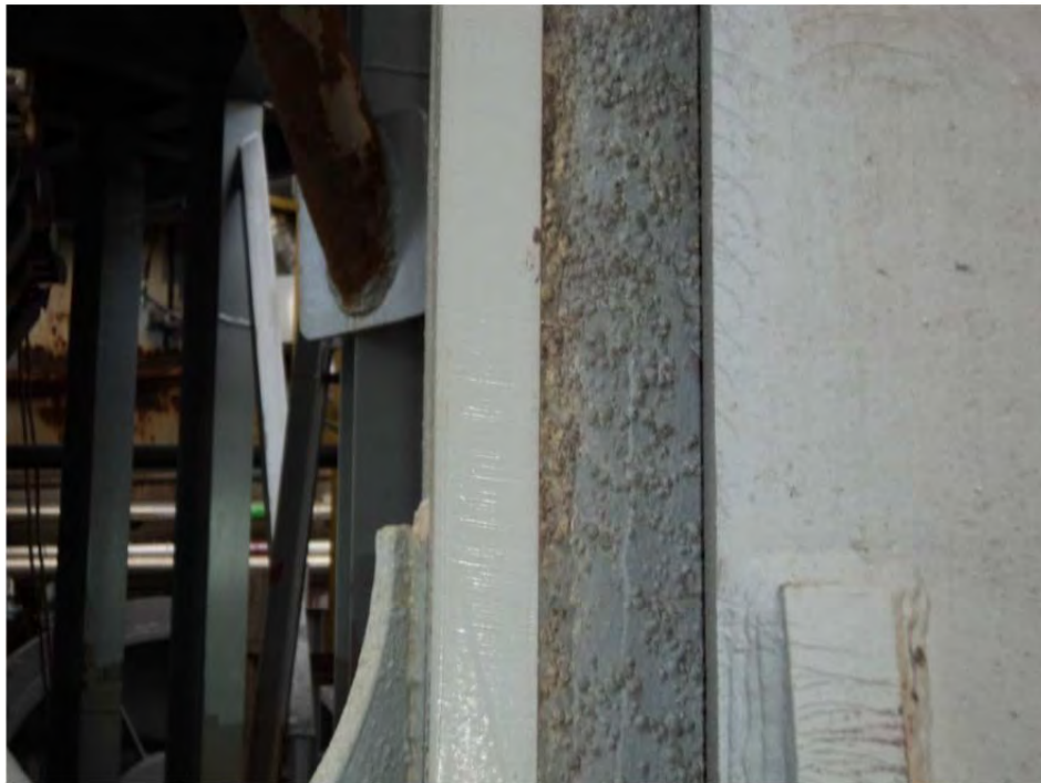
Photo 2. Dead barnacles shell on Starboard Leg (left) at the jacking guide slot on the right. Most of the barnacles have been painted over during the latest painting of the legs (gray paint).
