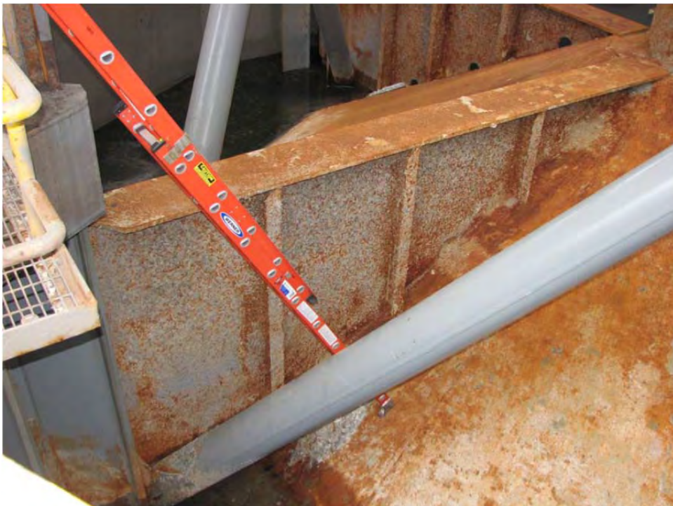
Photo 14. Encrusted marine organisms (grayish film) on spud can support member just above the water level on the Bow Leg.
