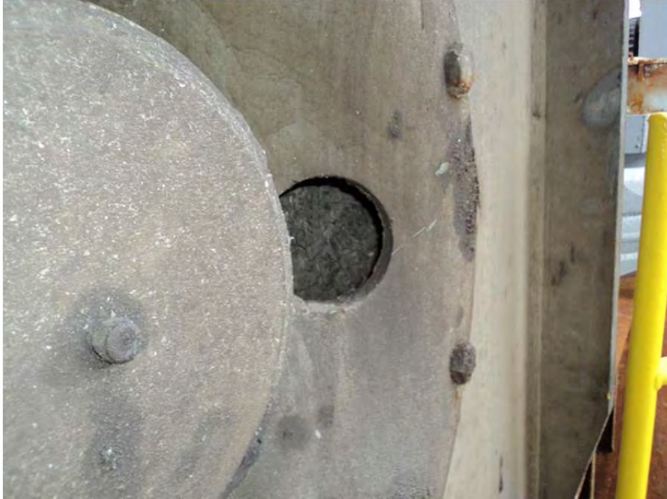
Photo 7. Old oyster shells on the inside the lower portion of the leg guide on D chord of the Starboard leg. Shells attached to this structure can only be seen through this opening when the legs are raised.
