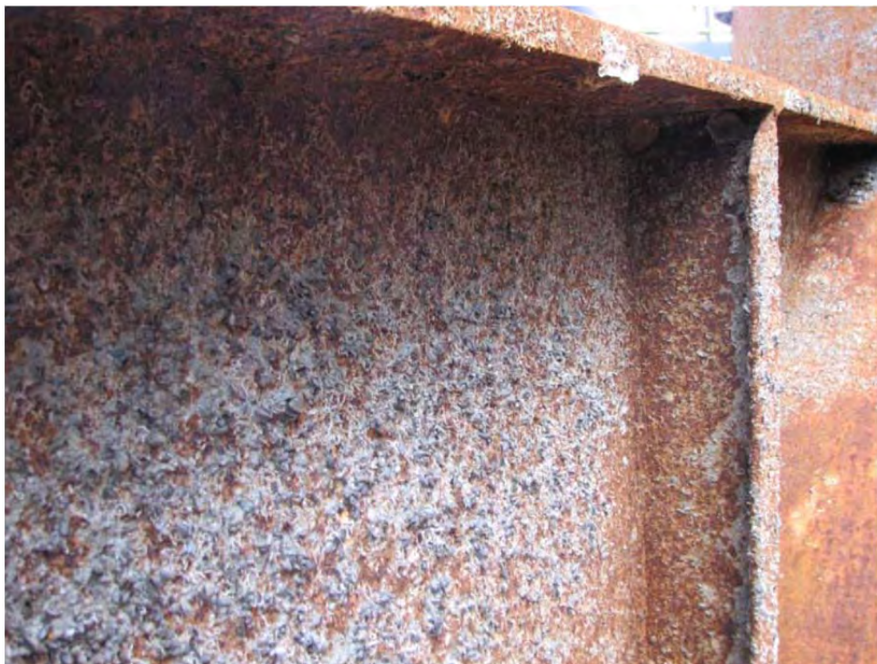
Photo 16. Close up of encrusted juvenile mussels and calcareous worm tubes on the spud can structural support member.
