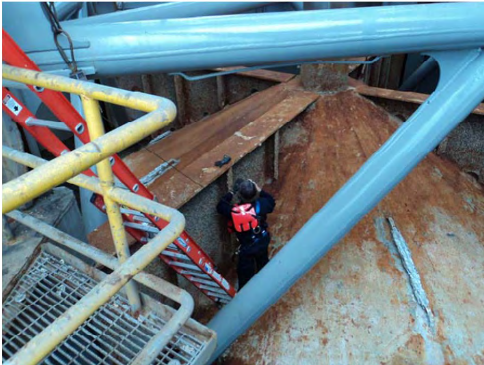
Photo 15. Worker preparing to take sample from vertical surface. Shell debris on the grate in the lower left.
