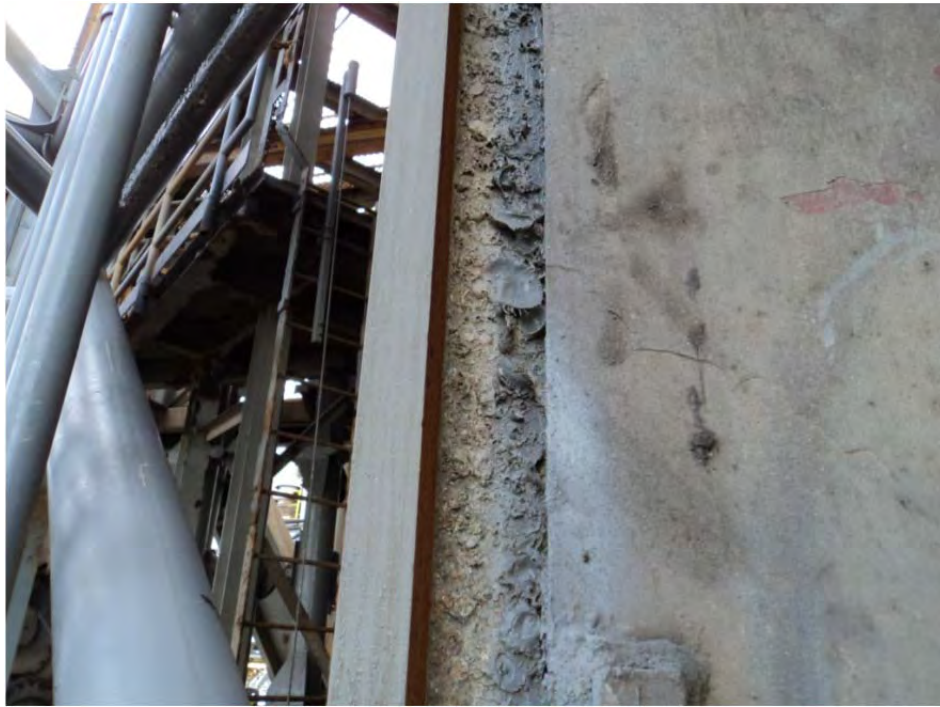
Photo 1. Old oyster shell on the bow leg (right) at the jacking guide slot (under gray paint). Operation of the jacking mechanism doesn't remove the old shells.
