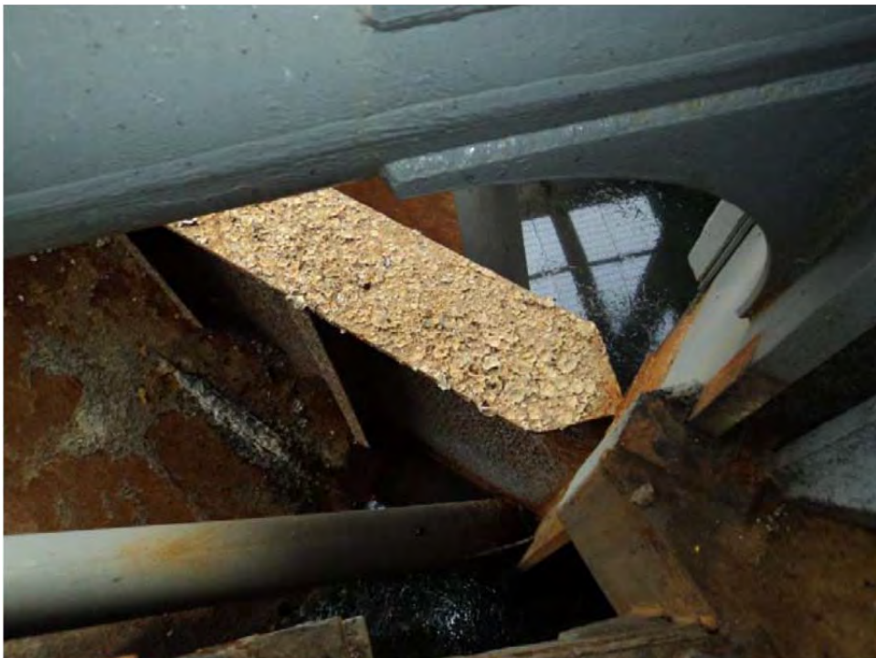
Photo 4. Old oyster attachments on the top of a support member on the spud can. No live oysters
