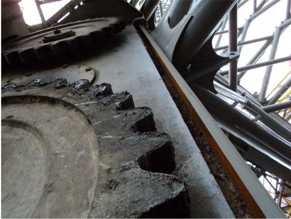
Photo 3. Old shells encrusted on the Bow Leg in the slot by the jacking guide. Shells extend up to the next deck level.
