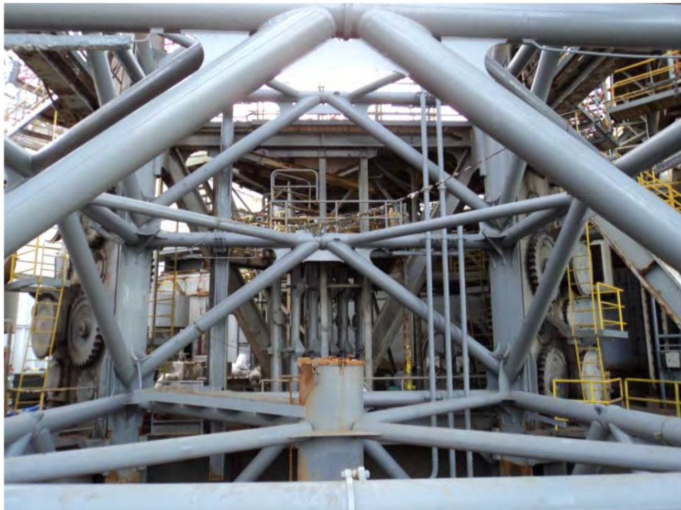
Photo 6. Cable stretched across bow leg (center of photo) with encrusting marine organisms. This cable was likely underwater when the rig was cold-stacked.
