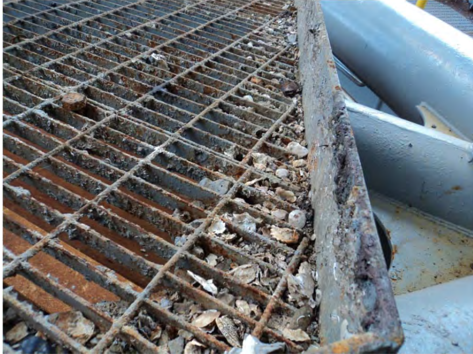
Photo 5. Shell debris on the catwalk out to the manhole on top of the spud can. Debris likely collected from cleaning the legs of encrusting marine biota prior to painting the legs.
