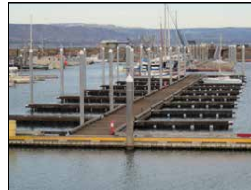
System 1 float replacements and upgrades.
