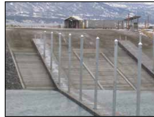
New load and launch ramp completed in Dec. 2015.
