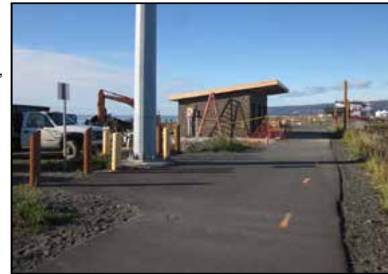
New restroom and trail additions to Homer Harbor.
