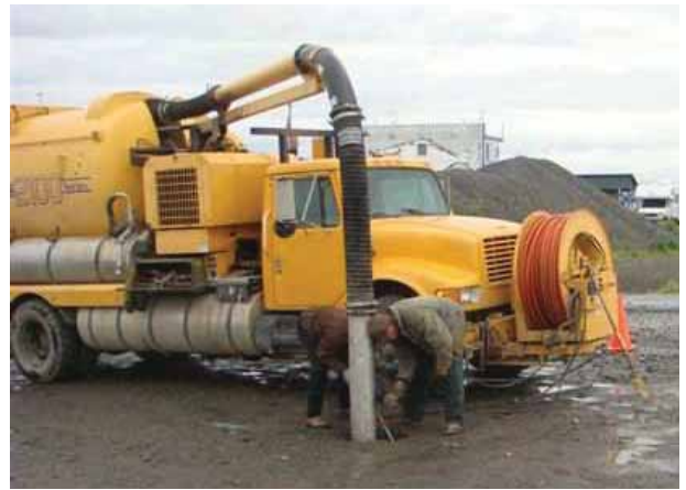
Rick Klopp and Rusty Cheney operate a vector truck as part of a dredge spoils dewatering project on the Homer Spit.
