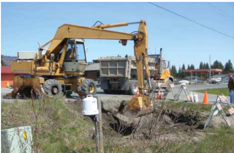
A Public Works crew repairs a water line on Ocean Drive.
