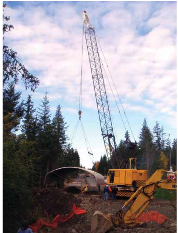
A crane prepares to move part of the Woodard Creek bridge into place to complete Spruceview Avenue. The project included a separated trail.
