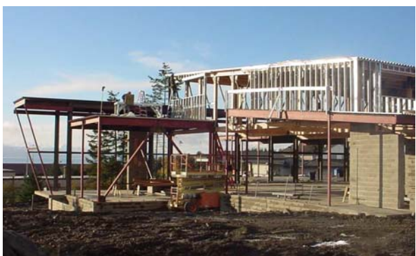
New library under construction, October 25, 2005.
