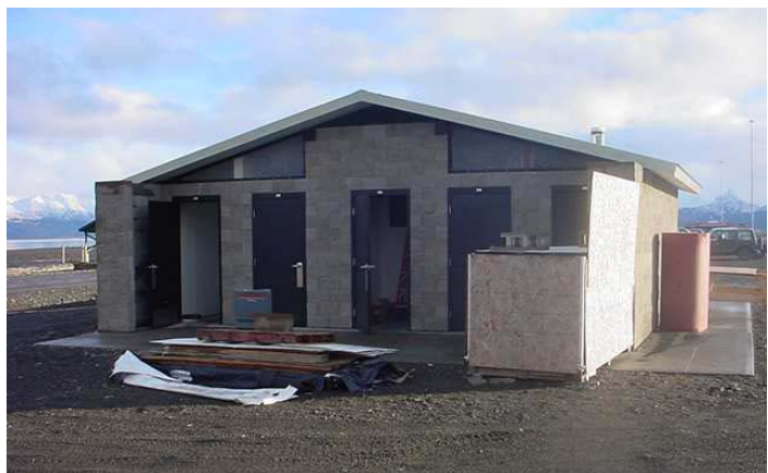
Residents and visitors alike were happy to see construction of a new restroom at Ramp 4 of the Homer Harbor.
