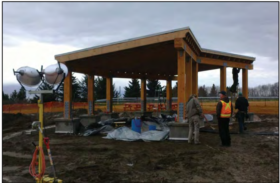
New pavilion at Karen Hornaday Park mid construction.
