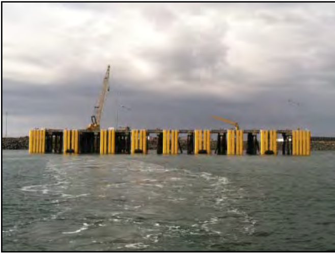
New fenders were installed on the Deep Water Dock in 2013.
