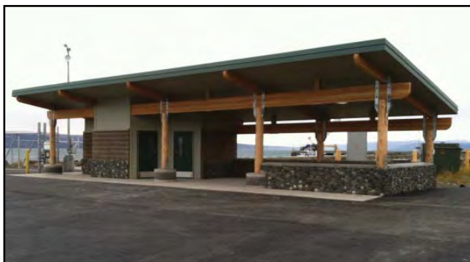
Guard shack and restroom at the Deep Water Dock.
