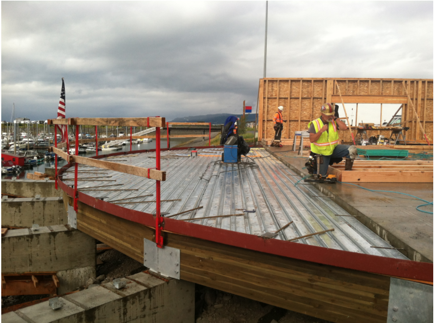
New harbormaster office, under construction
