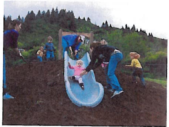
Families First funded a new slide and boulders for Bayview Park and organized a work party to install equipment and perform other safety maintenance with the Parks & Rec Department (May 2011).
