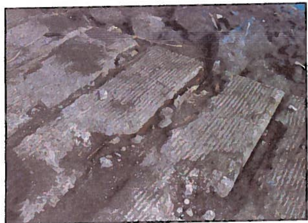
Load & Launch Ramp Deterioration
