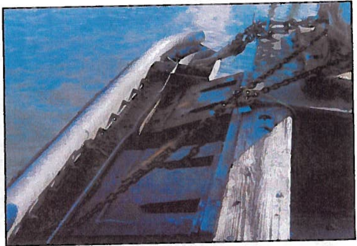
Deep Water Dock – Missing fender & fender being held on by chains
