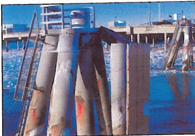
Pioneer Dock Damaged Dolphin
