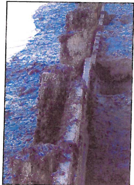
Corrosion on Pioneer Dock and Fish Dock Pilings
