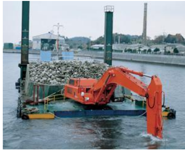
Figure 7: Dredge Barge with Excavator for cleaning Channel; similar to the cradle mechanism the for barge option. Retrieved from www.hcmm.com.my .
