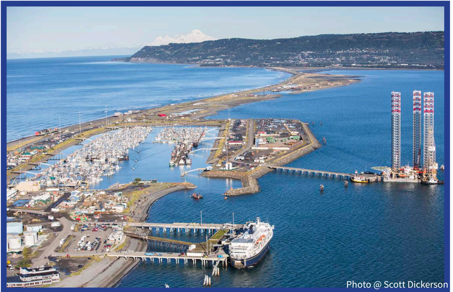
This aerial shot of the Homer Harbor shows a Port town hard at work with the Alaska State Ferry Vessel Tustumena in port, the jack-up rig Endeavor at the Deep Water Dock and boats coming and going through the mouth of the harbor.
