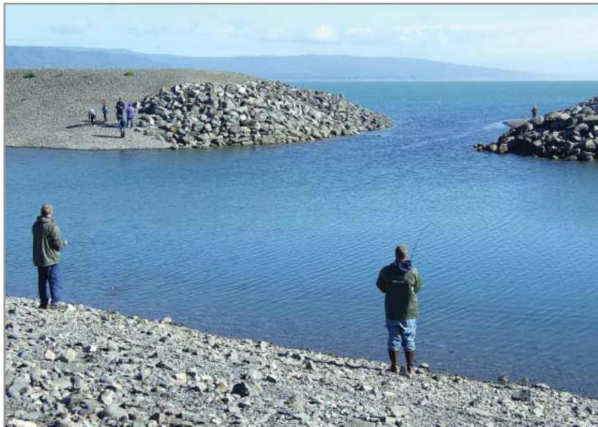
Significant improvements were accomplished at the Fishing Lagoon in 2010, including removing a gravel bar that had formed at the north side of the entrance and rebuilding the north berm with armor rock. Additional dredging work is needed now.
