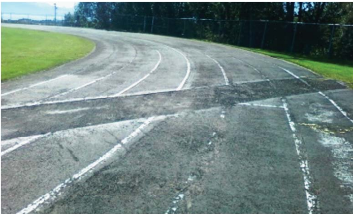
Left: The area of the track that was patched after the 2002 floods is not level.
