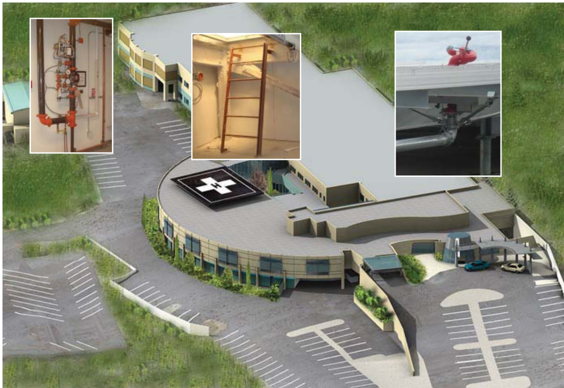
Architectural drawing of completed project with insets of work completed to date to accommodate the AFFF Foam Suppression System.
