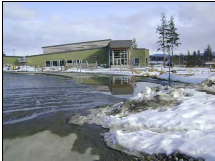
A master plan is needed to address storm water management issues. This picture of the Homer library parking lot is an example of flooding and overflows that occur community wide during rain storm events.
