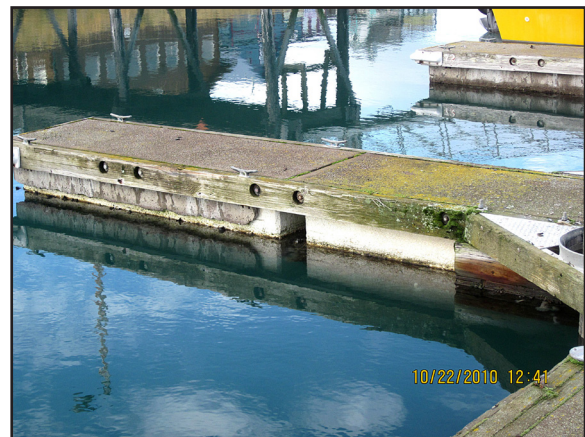
Exposed flotation on a damaged float.
