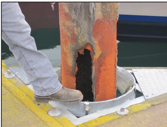
Hole in damaged piling that needs replacing
