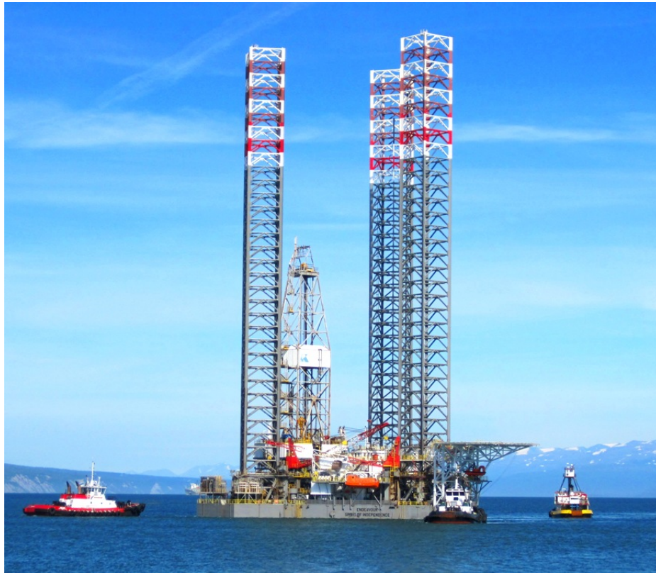
Figure 1. Buccaneer’s ‘Endeavour – Spirit of Independence’ Jack-Up Drill Rig
