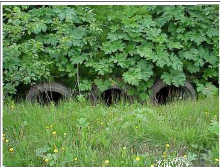
Storm Drains on Sterling Highway Draining to Bay
