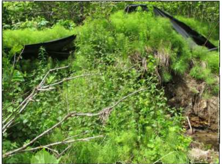
Failing erosion controls viewed at upper end of reach at KB-180, right bank, June 2012.
