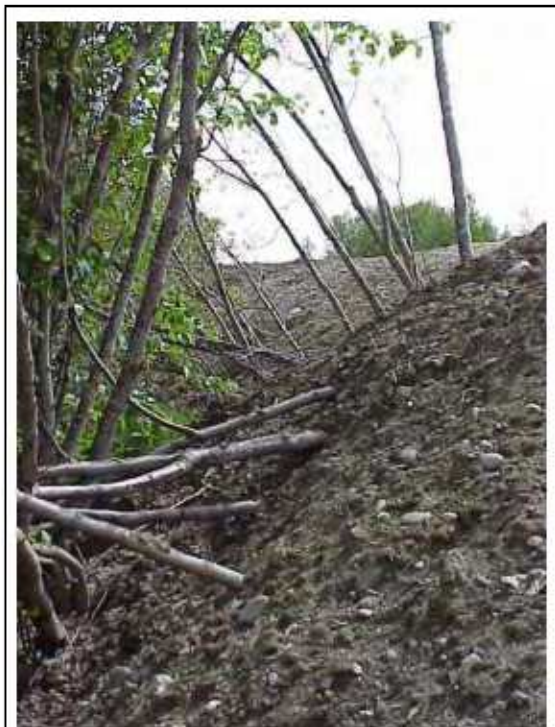
Fill pushed into streambank at Hornaday Park
