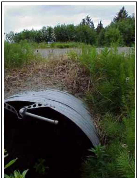
Culvert and Paved Lot along Pioneer Avenue
