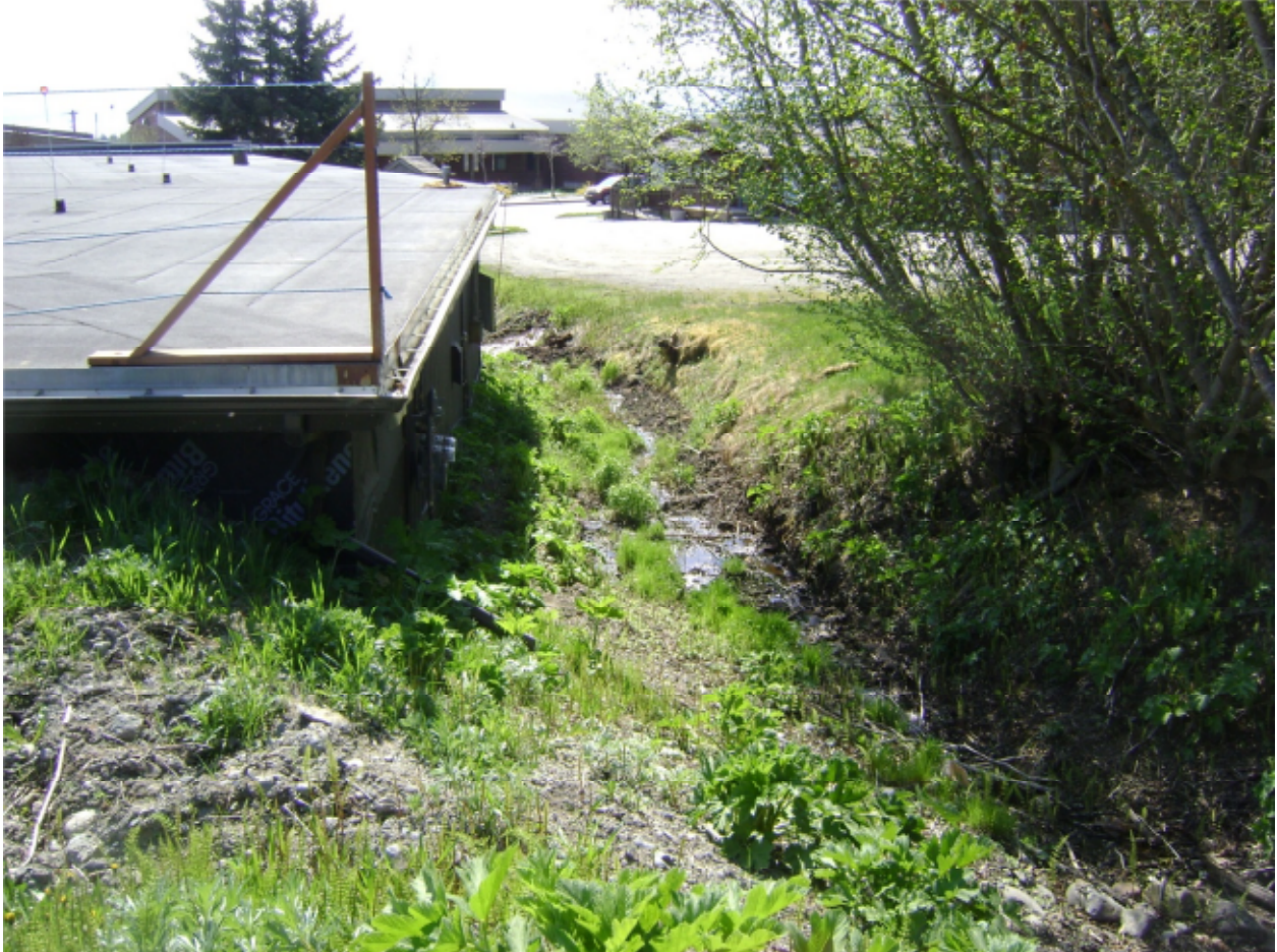
Northwest corner of the building. There is a ditch to the west that runs down between the properties.
