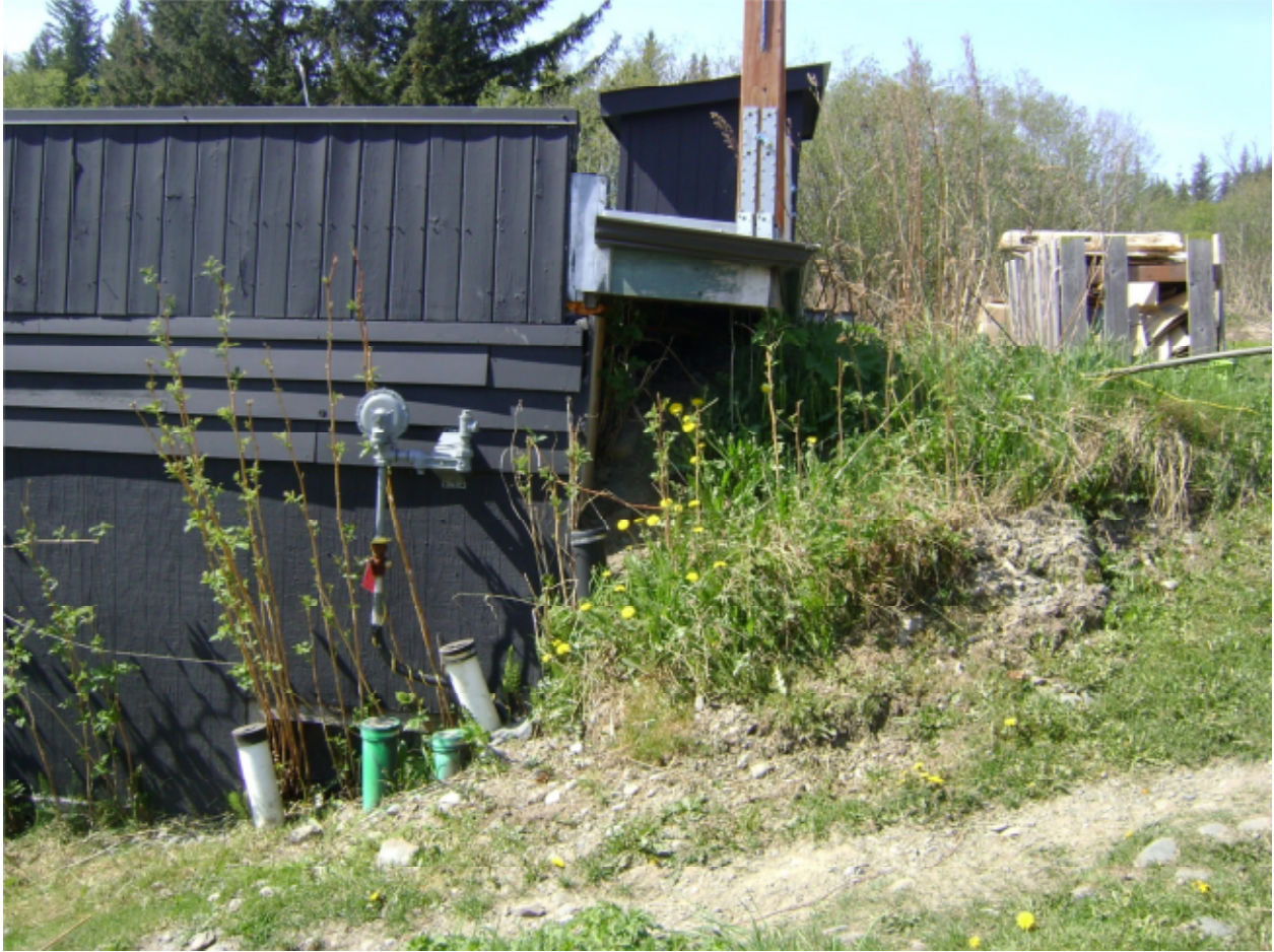
Northeast corner of the building. Notice back fill up to about roof level. The crate to the right appears to be a recycle/storage area for cardboard.
