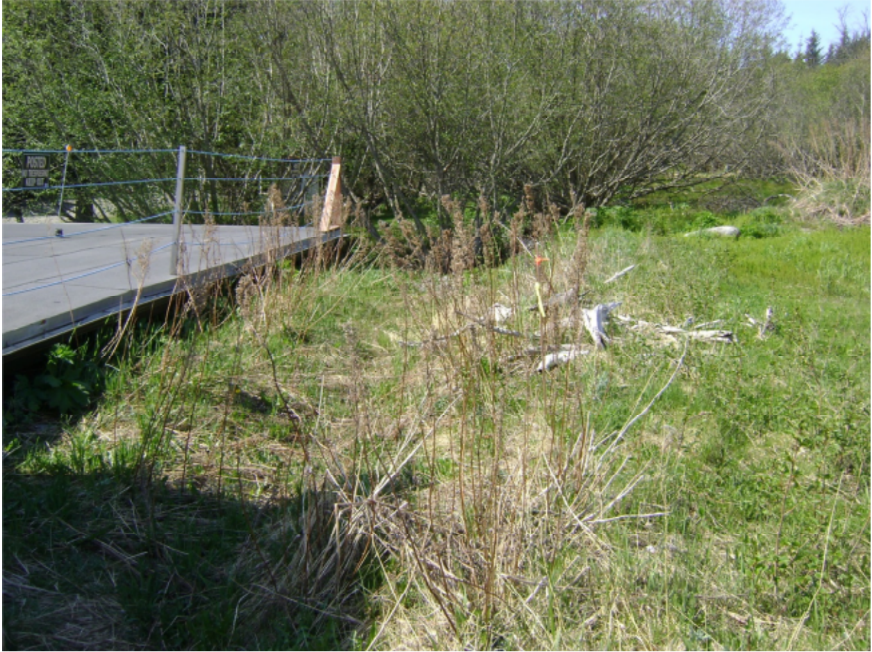
Northwest corner of the building, standing on Lee Drive ROW. There is a stake in the photo although staff did not verify what it was marking. There is a ditch between the road elevation, and the back of the building.
