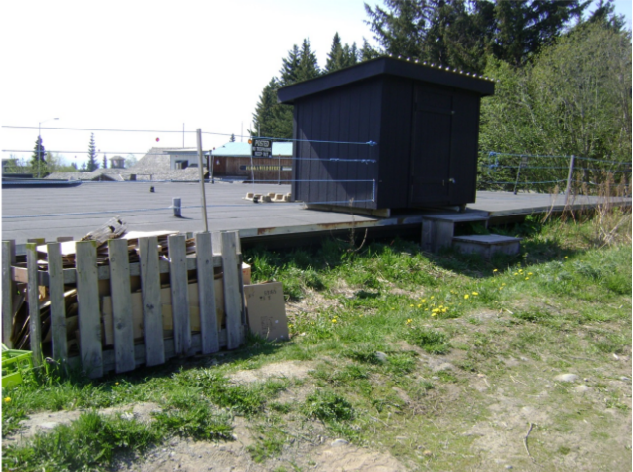
Standing on Lee Drive looking southwest over the building roof. There is what appears to be cardboard/shipping material recycling on the right. There is a storage shed on the roof. Public access to the roof is controlled by a rope fence along the perimeter of the roof.
