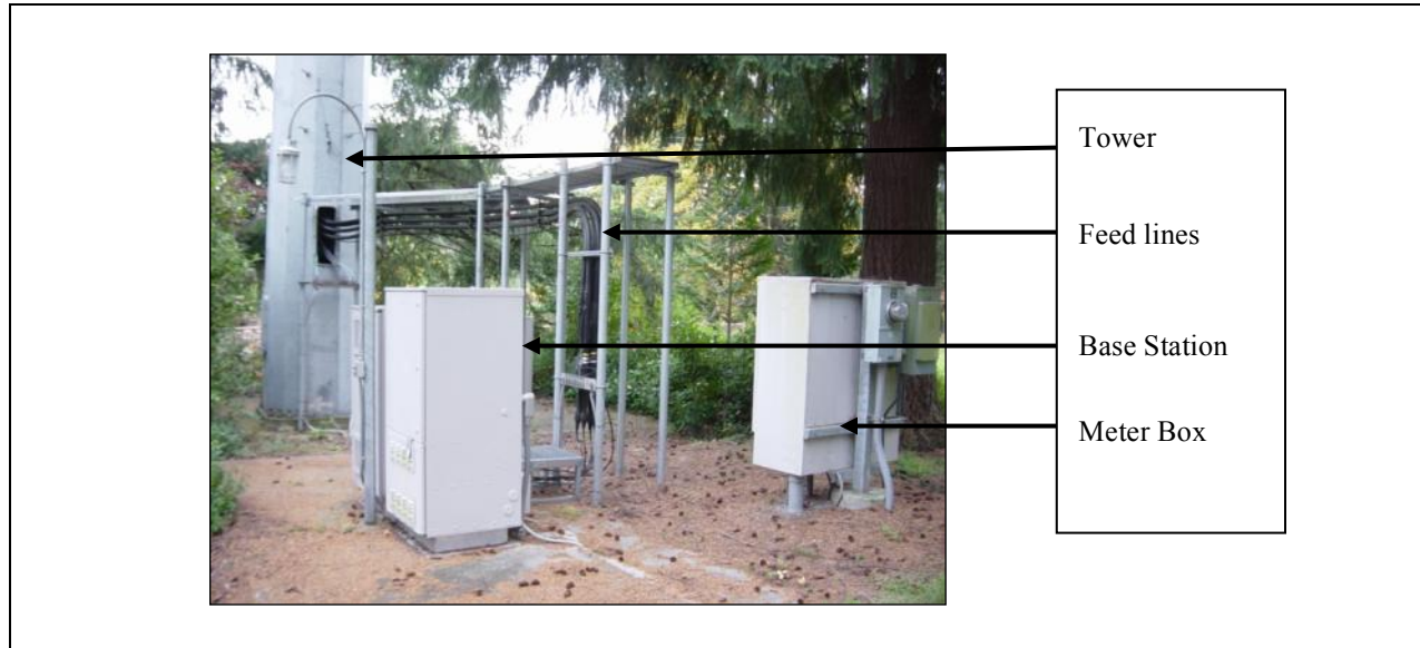
Figure 1: Example of 1900 MHz Wireless Infrastructure Ground Equipment
