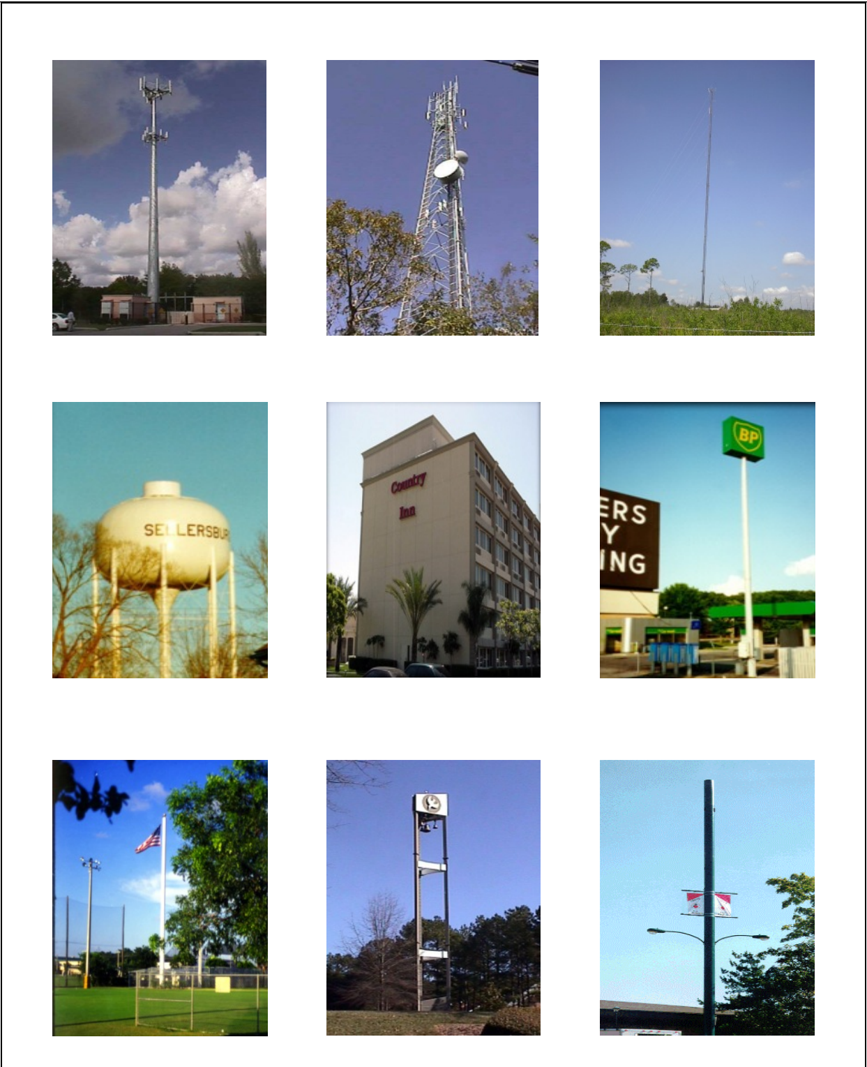
Figure 5: Examples of Antenna Support Facilities
