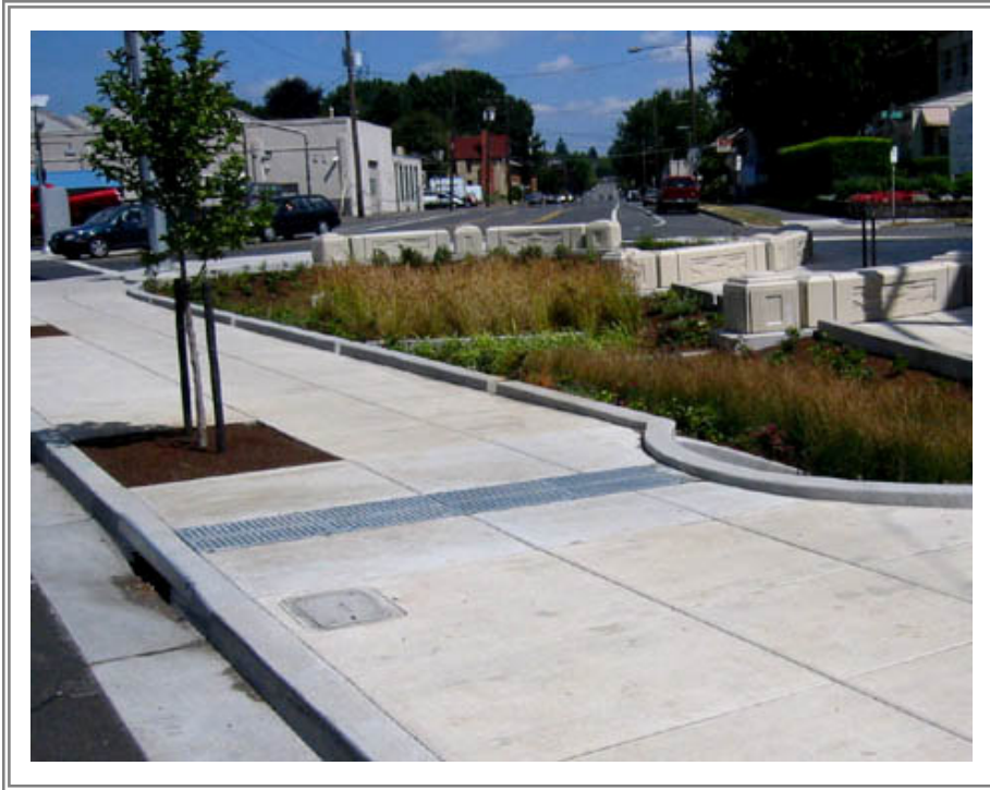
Figure 8 - Curb and gutter directing runoff to a rain garden in Portland, OR
