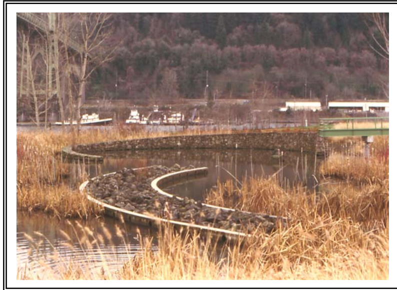
Figure 10 - Portland Pollution Control Lab – pipe and pond
