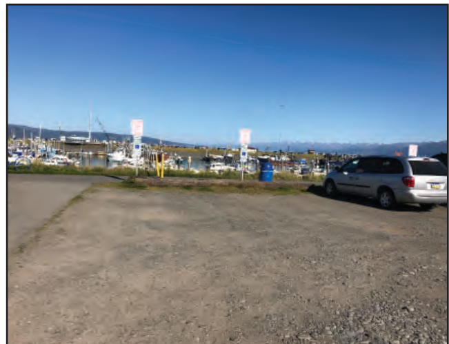
While inaccessibility issues in these spaces has been remedied since this photo was taken, it provides an example of spaces needing to be paved and a path of travel to the sidewalk provided .
