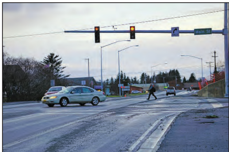
HAPP completes important sidewalk connections and installs high visibility crosswalks to improve non-motorized transportation and safety..
