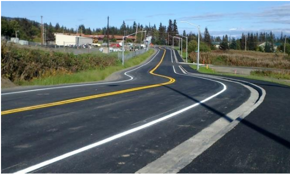
Waddell Way Improvements
