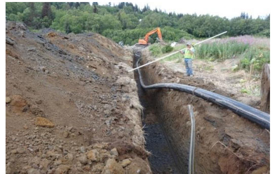
Shellfish Avenue Water Main Installation
