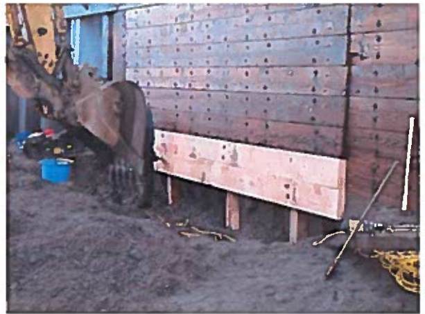
Lower wall repair - 2011
