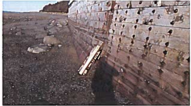
Timber face damage - repaired in 2016
