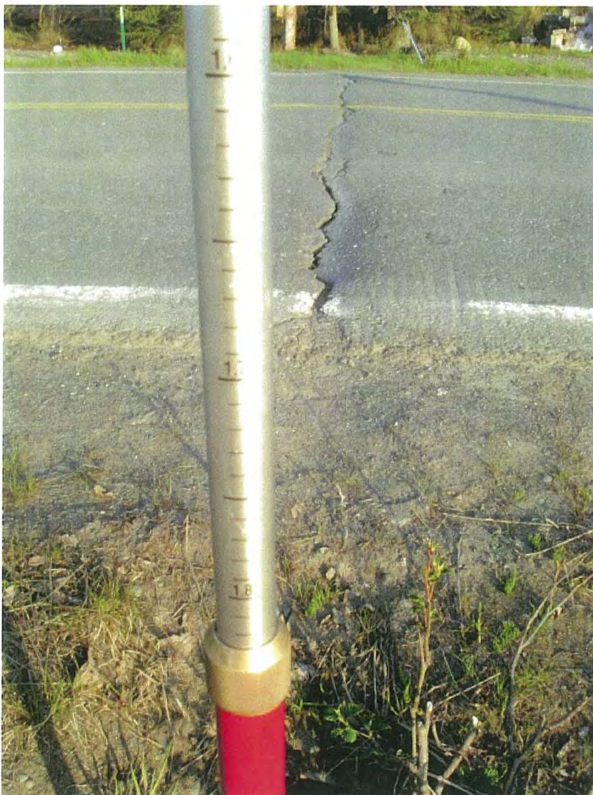
Photo 4: Road Surface Crack Separating Area Between Photo 2 and Photo 3, At Location of Photo 2 (Kachemak Drive), 2008
