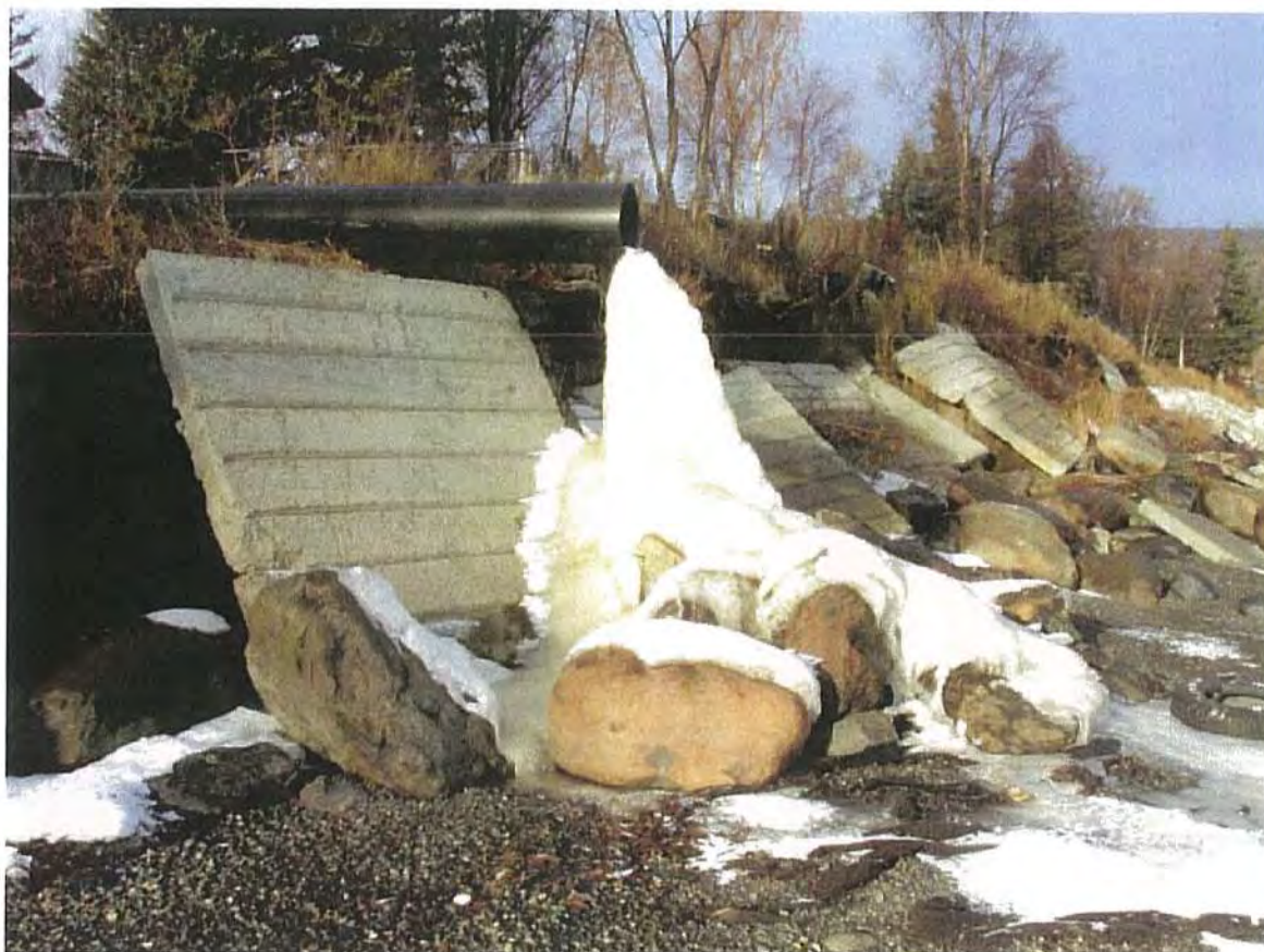
Photo 4. Kachemak Drive Bluff Discharge from Surface Water
