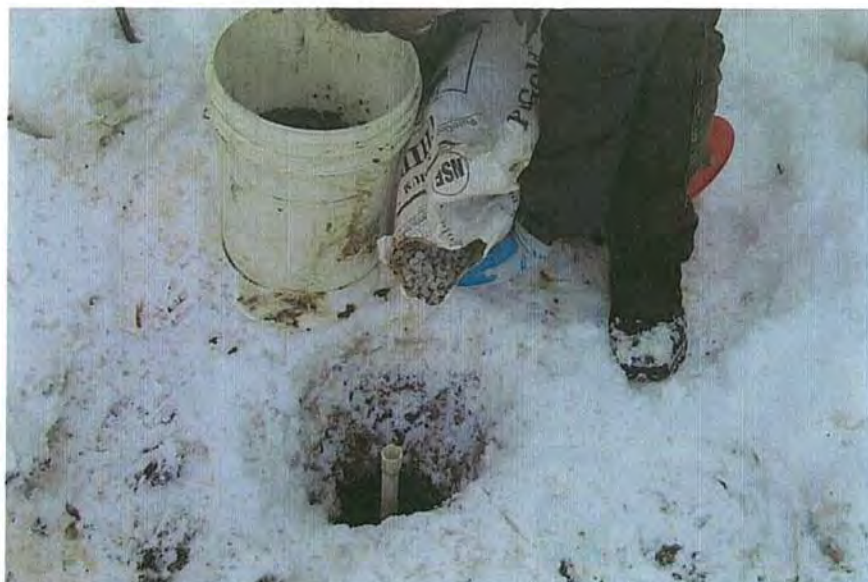
Photograph E. Winter Installation of Piezometer; Bentonite Seal, 2/4/04
