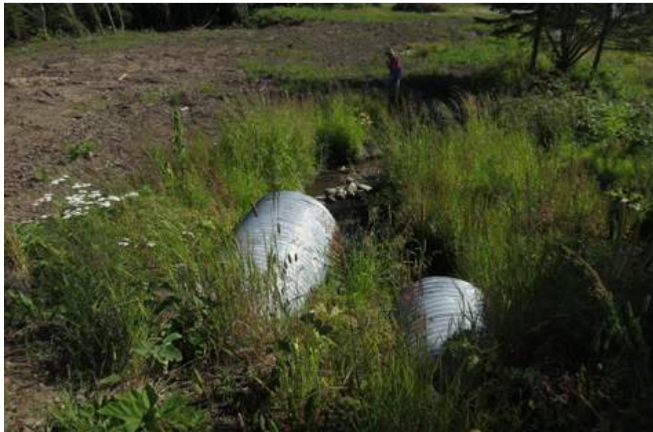
Pioneer Avenue culvert outlet. Source: Lisa Holzapfel.
