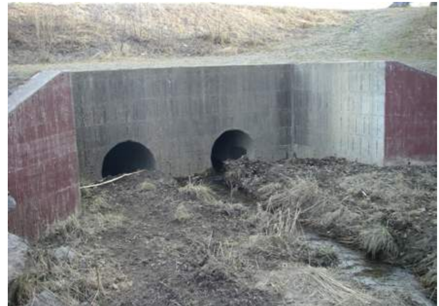
Fairview Avenue culverts. Source: Bill Spencer.
