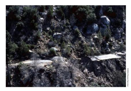
**Figure 7-8.** Landslide damage to Stump Springs Road on the Sierra National Forest, California. Note large rocks from rockslide onto the road in the background. This is one of thirteen damaging landslides from precipitation events affecting the Sierra Nevada in 1982 and 1983.
