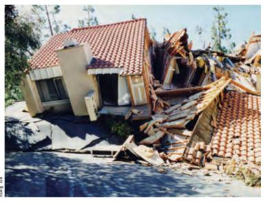
**Figure 7-2.** Street view of damage caused by the Laguna Niguel landslide. Such occurrences have been the driving force for the development and evolution of grading codes in California.
