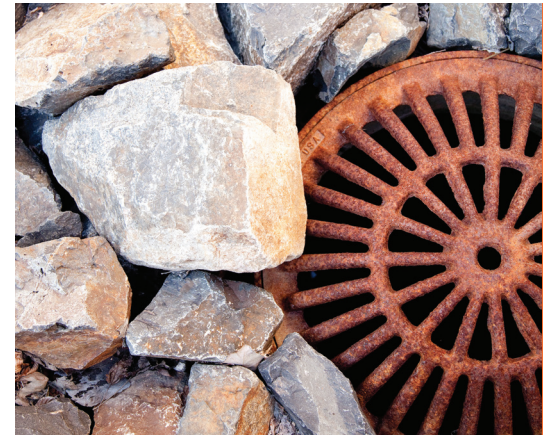
The Brewery, infiltration trench, Milwaukee
