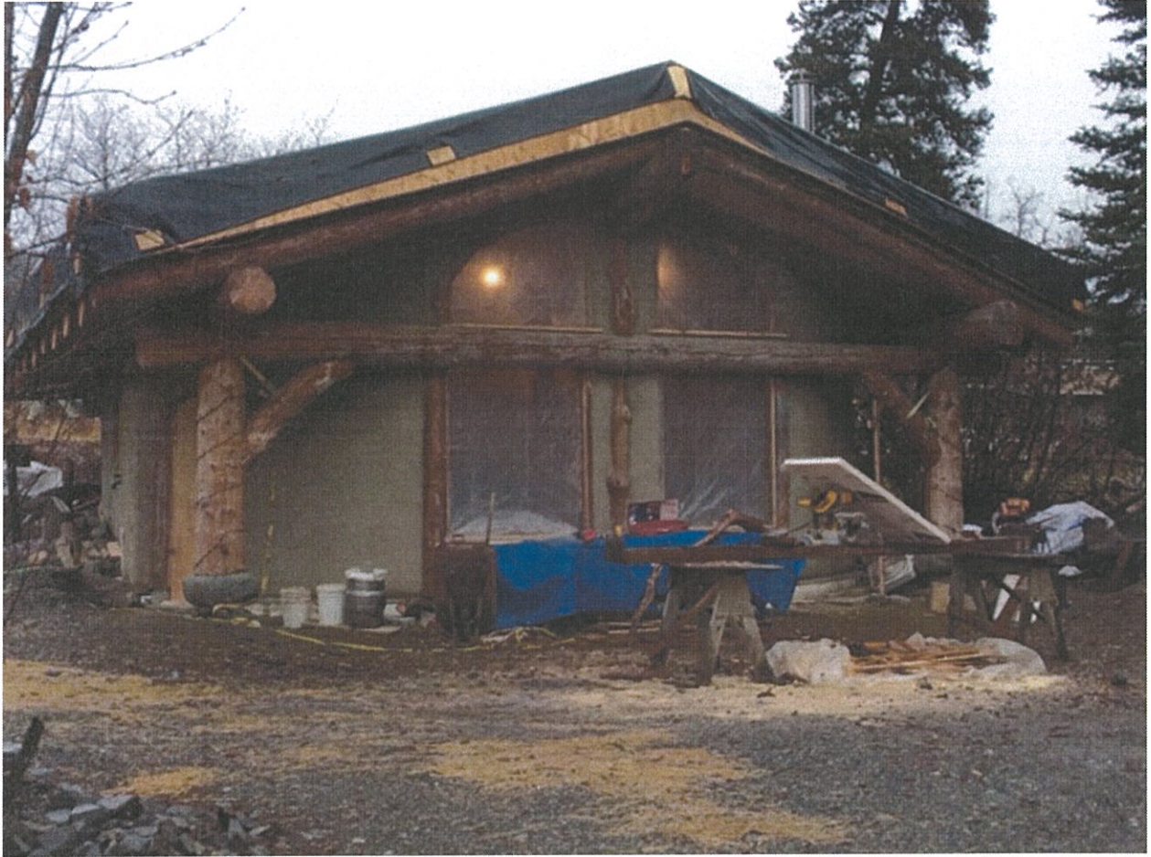
Cottage. Similar concrete or stucco type siding to the utility building. The siding looked very fresh during the site visit as if recently completed or in the curing stages.
