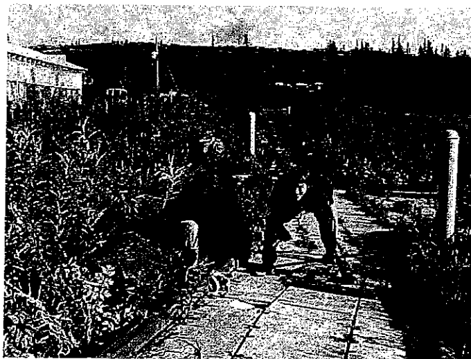
The Beluga Slough Trail has been plagued with problems and is difficult to repair. Some parts of the original trail are missing altogether.
