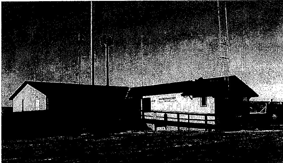
The current Port & Harbor building has never met codes for occupancy as an office building.
