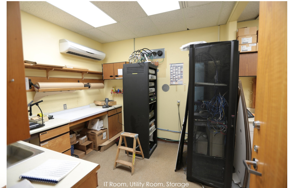
IT Room, Utility Room, Storage
