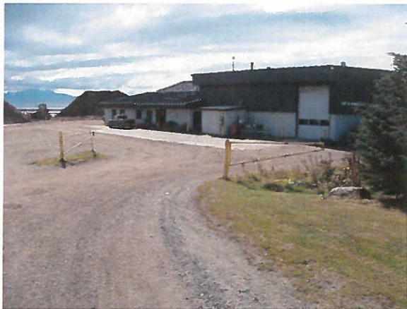
Existing Public Works building
