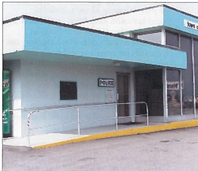
A town chose to alter its police station rather than move its programs and services to another accessible location.
