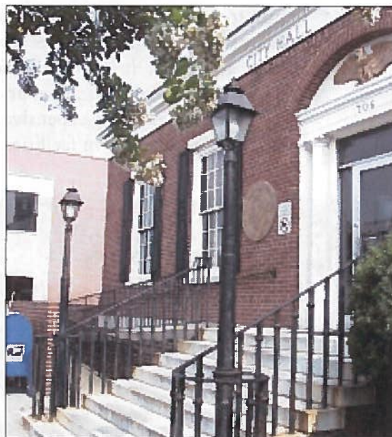
A ramp located next to the stairs to this town hall provides an accessible entrance.
