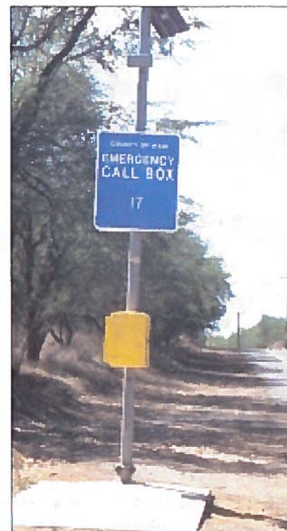
An emergency call box located in a rural area is mounted in an accessible location and can be used with or without speech to provide effective communication.
