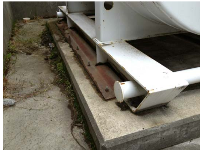
EXISTING FUEL TANK AND SLAB WITH SKID CLAMP
