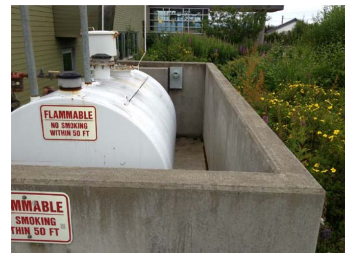
EXISTING TANK AND ENCLOSURE LOOKING SOUTH
