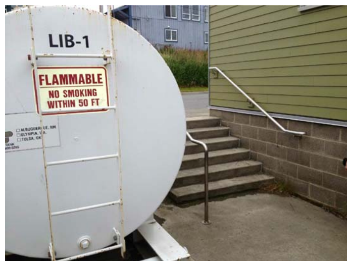
EXISTING FUEL TANK AND STAIRS
