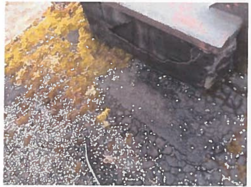
Hatch access on Tank Roof
