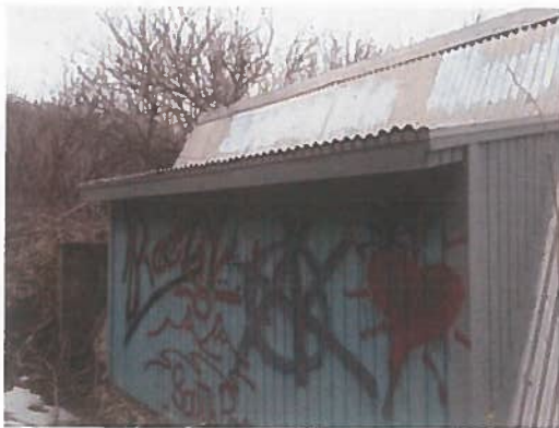
Mechanical Bldg side view
