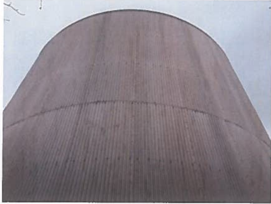
Water Tank View
