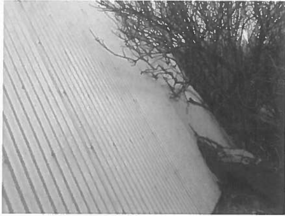
Mechanical Bldg Roof
