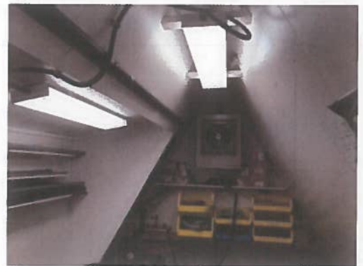
Interior Mechanical Bldg
