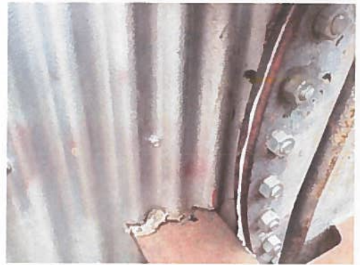
Gasket and Black Caulking
