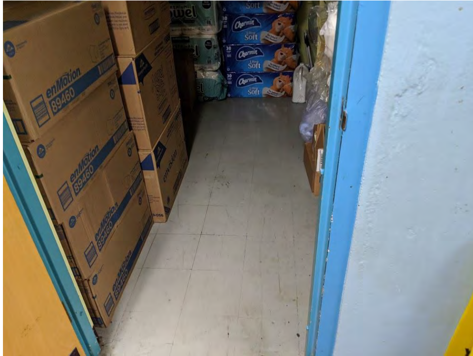
Photo 23: This photo shows ACM grey floor tile and black mastic under the floor tile in the storage closet.
