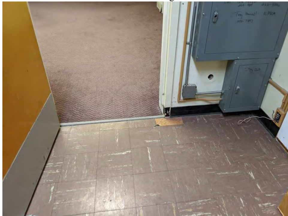
Photo 14: This photo shows ACM black mastic under the floor tile in the storage closet of the fan room.
