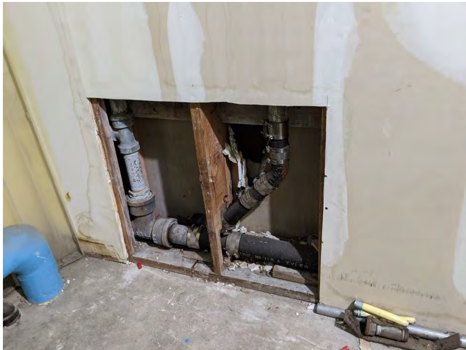
Photo 18: This photo shows ACM tan joint compound attached to plywood in one wall found in the fan room.
