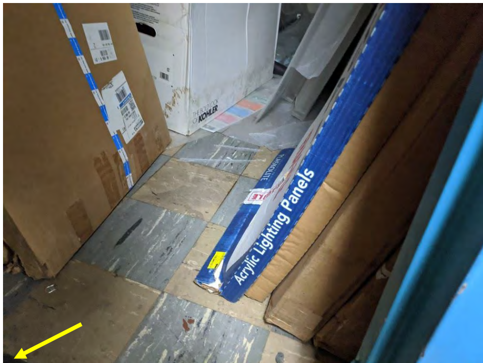
Photo 28: This photo shows sample location HERC 2-018 which is of ACM grey/yellow floor tile and black mastic under the floor tile found in the storage closet.
