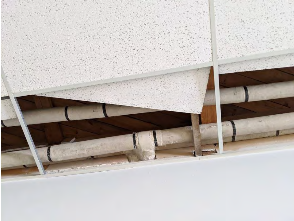
Photo 7: This photo shows the location of ACM off-white wrap around a pipe elbow found in the ceiling of room 111.
