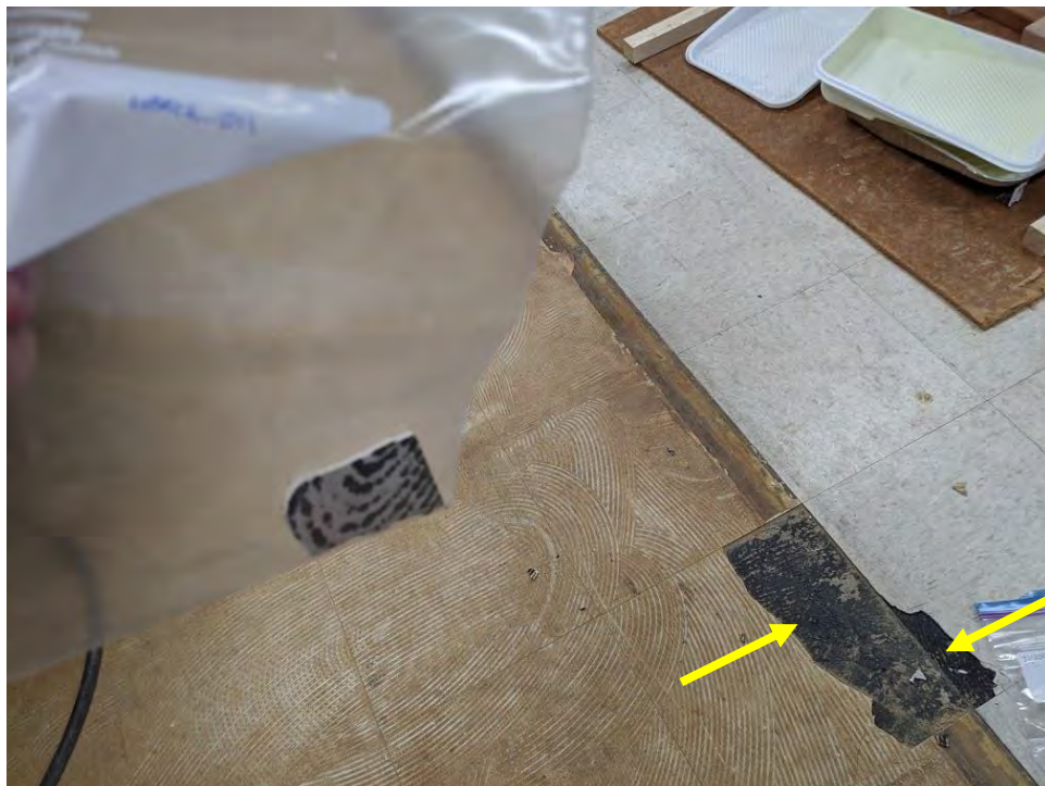
Photo 26: This photo shows sample locations HERC 2-011 and 012 which is of ACM black mastic under the floor tiles found in classroom 1.
