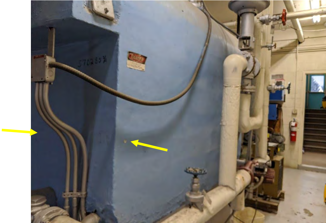
Photo 29: This photo shows sample locations HERC 2-021 and 022 which is of ACM white insulation coating a boiler found in the boiler room.
