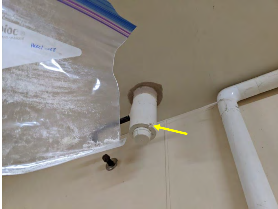
Photo 19: This photo shows sample location HERC 1-058 which is of ACM white insulation around a pipe found in the men's locker room.
