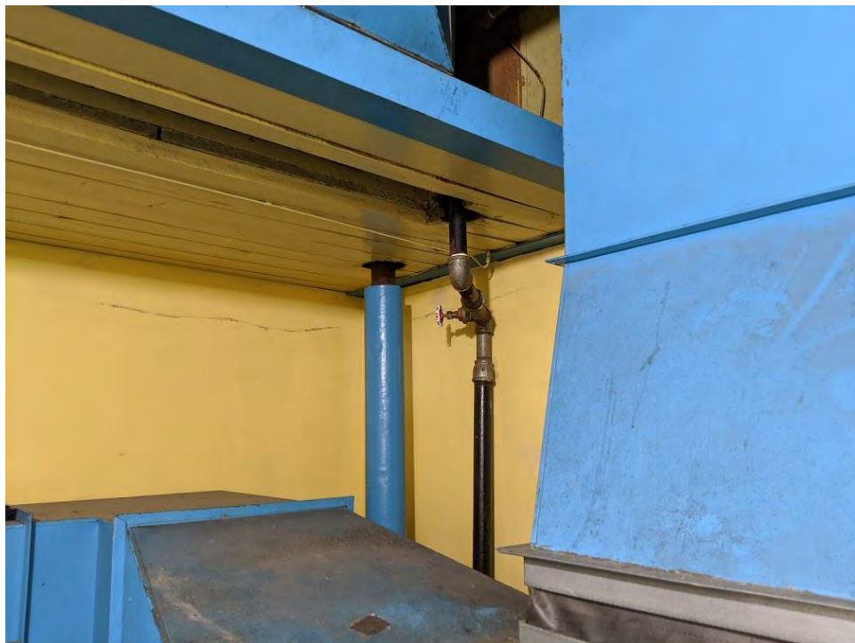
Photo 16: This photo shows piping that contained ACM off-white insulation around a pipe elbow found in the fan room.
