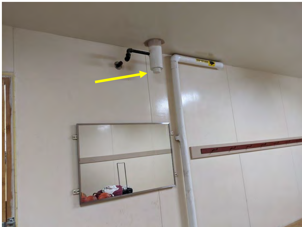
Photo 20: This photo shows ACM white insulation around a pipe found in the men's locker room.
