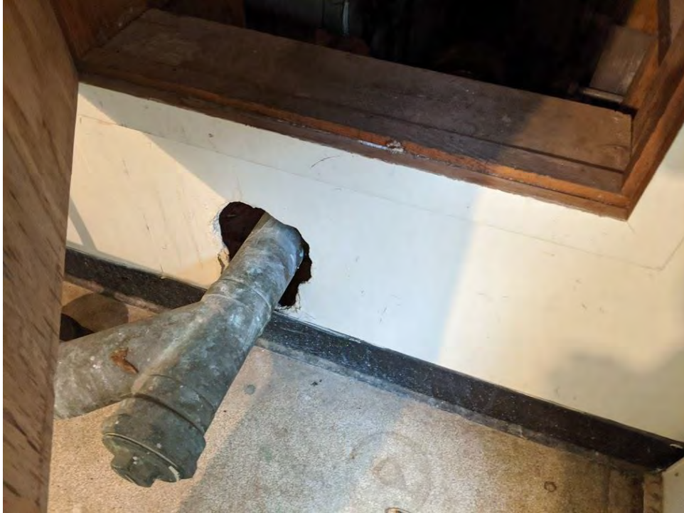
Photo 9: This photo shows protruding pipe into the wall in room 118 (janitor's closet between boy's and girl's restroom).
