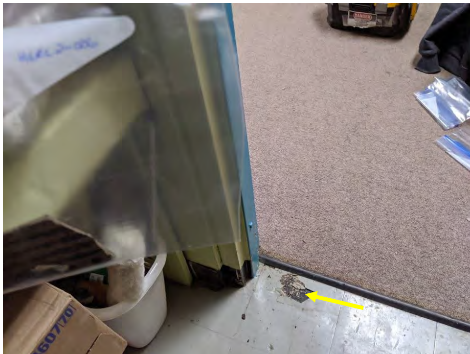
Photo 22: This photo shows sample location HERC 2-006 which is of ACM grey floor tile and black mastic under the floor tile in the storage closet.
