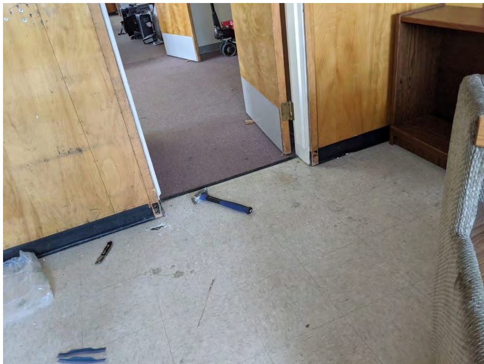
Photo 2: This photo shows ACM black mastic under the floor tile in room 107.
