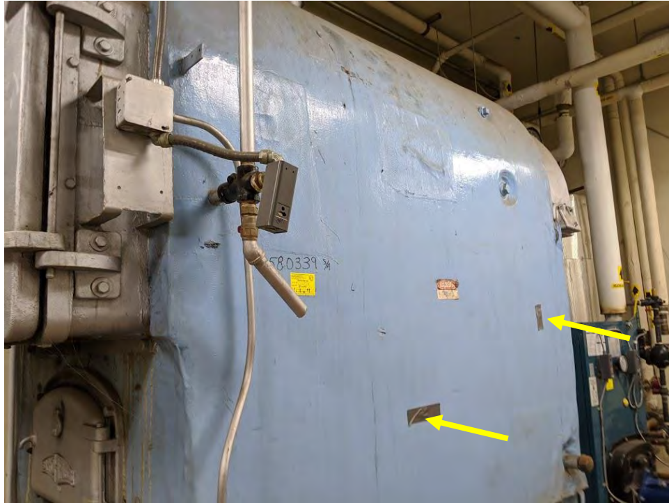
Photo 21: This photo shows sample locations HERC 1-064 and 065 which is of ACM white insulation coating a boiler found in the boiler room.
