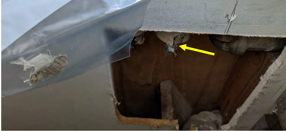
Photo 5: This photo shows sample location HERC 1-024 which is of ACM off-white wrap around a pipe elbow found in the walls of room 111 (science room).
