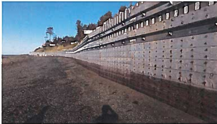
Sand/gravel build up protects toe of wall from erosion
