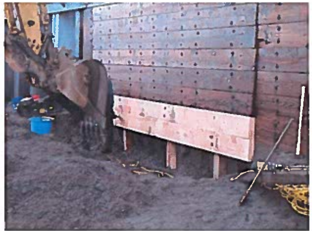
Lower wall repair - 2011
