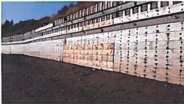
Repair made to panel section
