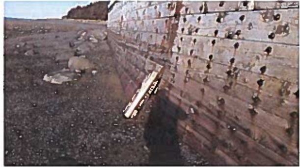
Timber face damage - repaired in 2016
