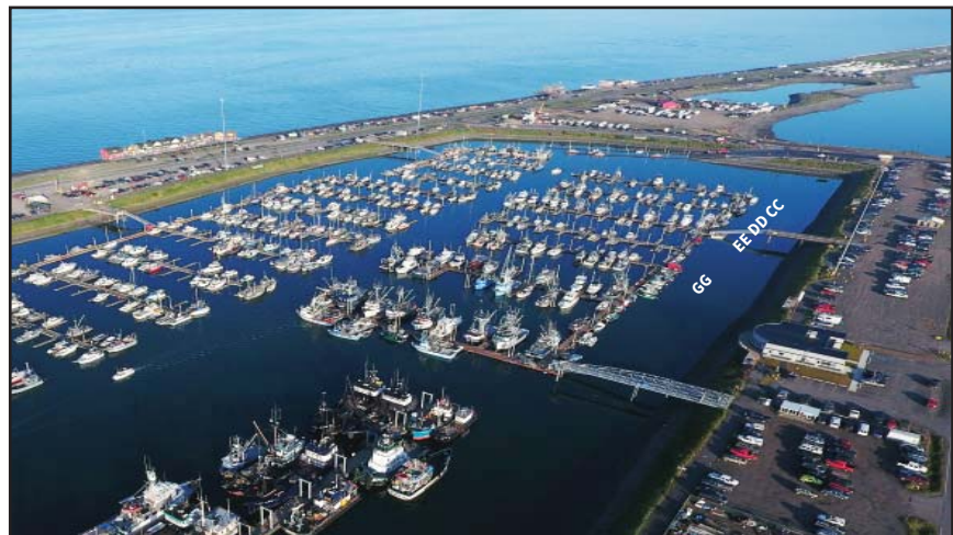
System 4 ramps to be replaced next.
