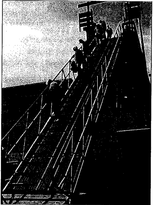
Ramp 3 is the most centrally located ramp in the Homer Harbor, but it is also the oldest and the most challenging to use at low tide. The old wooden approach to the ramp is also in need of replacement.
