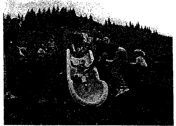
Families First funded a new slide and boulders for Bayview Park and organized a work party to install equipment and perform other safety maintenance with the Parks & Rec Department (May 2011).
