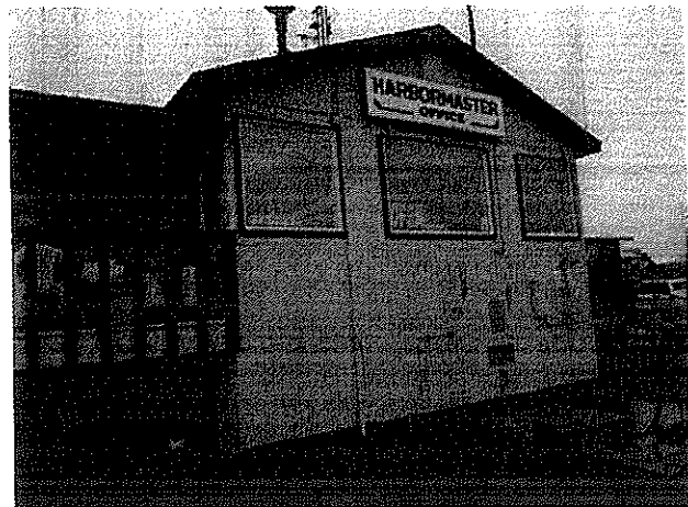
6. Harbormaster Office-North side.
