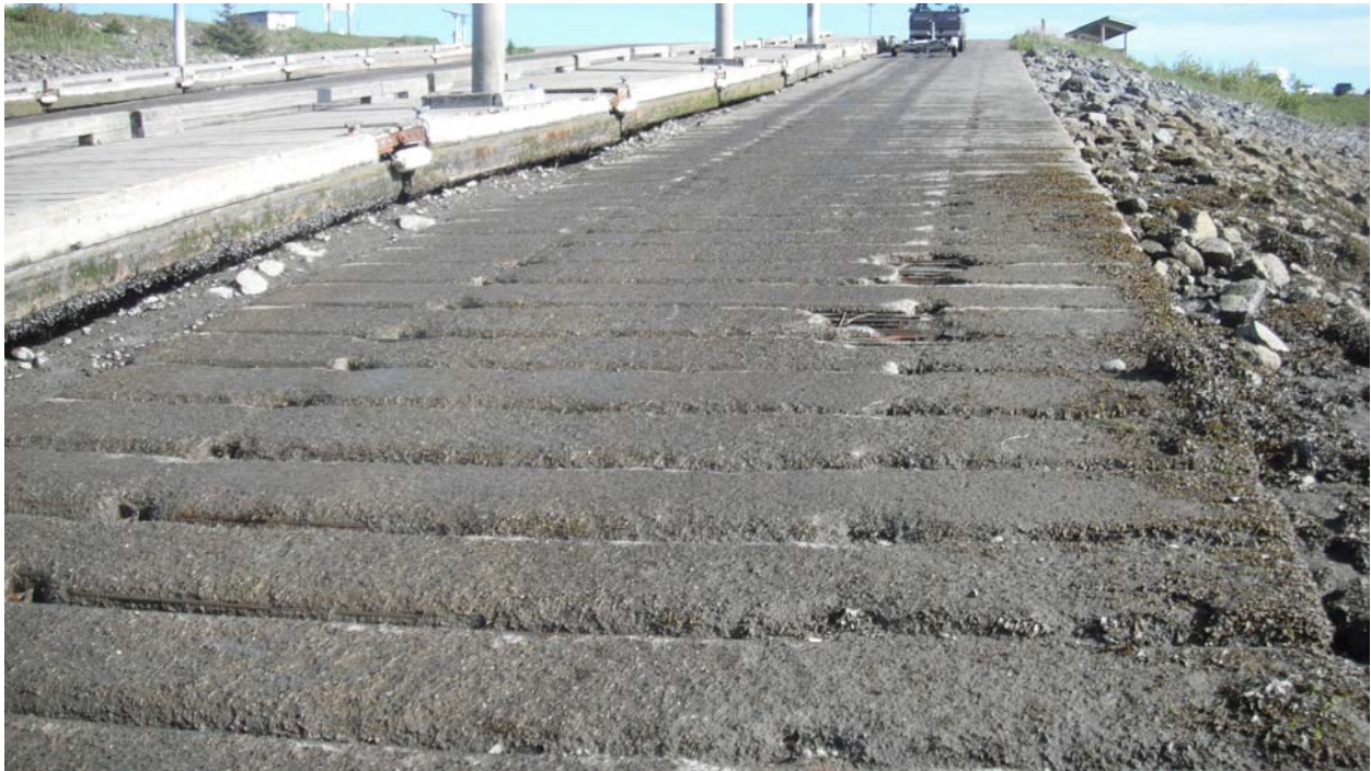
Figure 1-2: Existing Concrete Launch Planks
