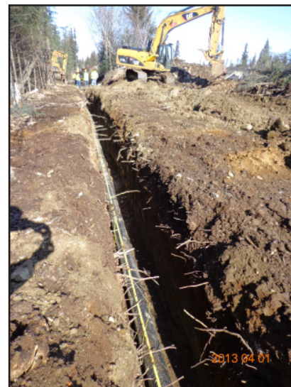
Enstar contractors trenching the trunk line.
