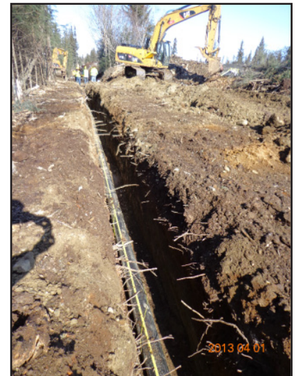
Enstar contractors trenching the trunk line.
