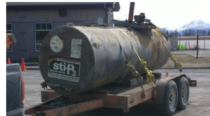
Airport Tank Removed
