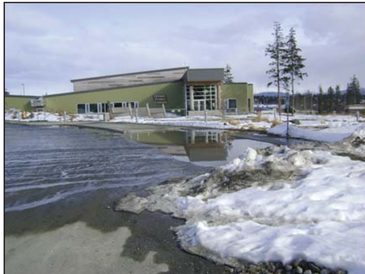
A master plan is needed to address storm water management issues. This picture of the Homer library parking lot is an example of flooding and overflows that occur community wide during rain storm events.
