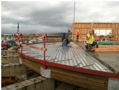
Harbormaster Overslope Construction
