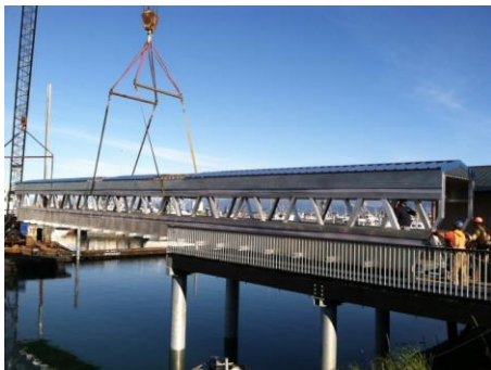
New Ramp 3 Being Installed
