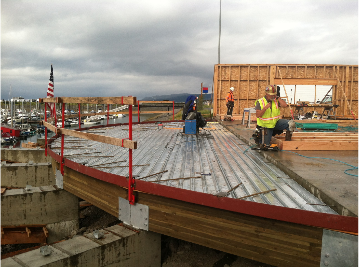
New harbormaster office, under construction
