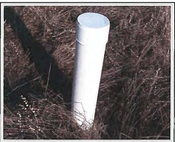
Sewer lines for additional cabins
