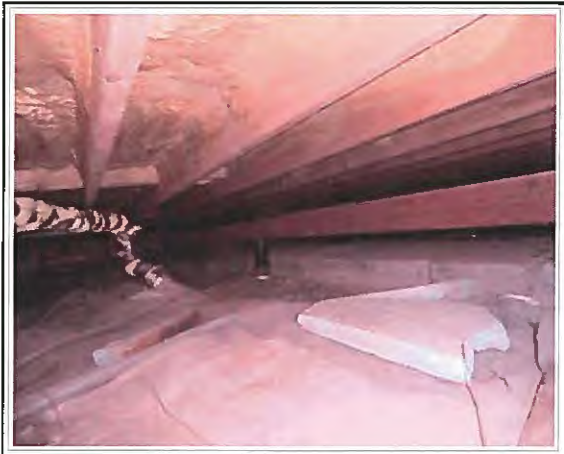
The underside of the floors have sprayed-in urethane foam insulation.
