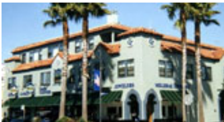
✚ Figure 5 Tower Disguised as Chimney
