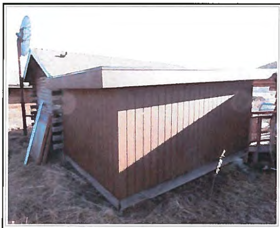
Storage shed (northwest side)
