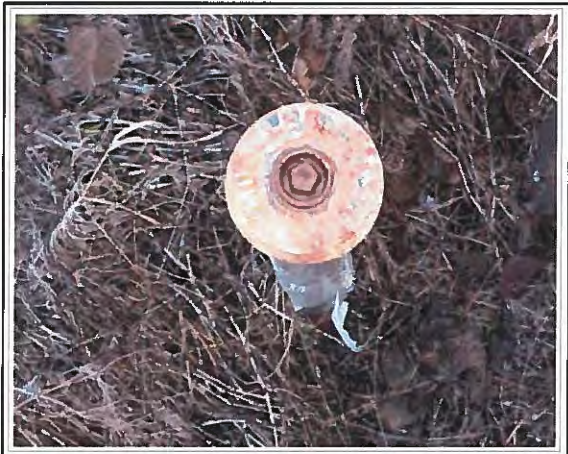
Each cabin has an individual curb stop for the city water line
