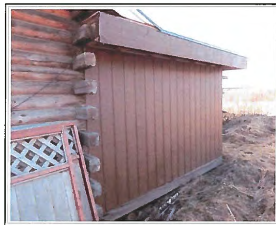
Storage shed (north side)
