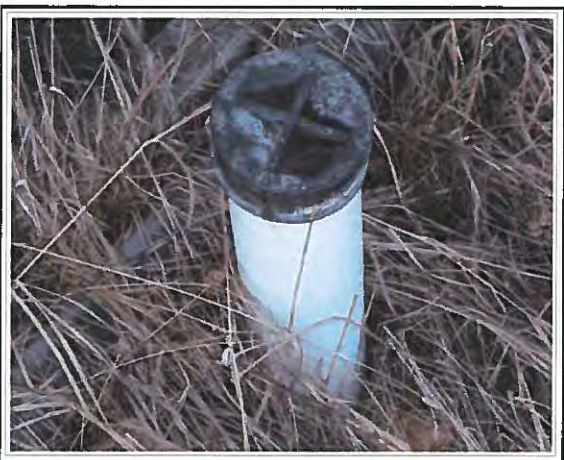
Sewer lines are stubbed in for two additional cabins
