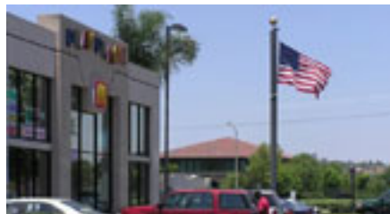
✚ Figure 6 Tower Disguised as Flag Pole
