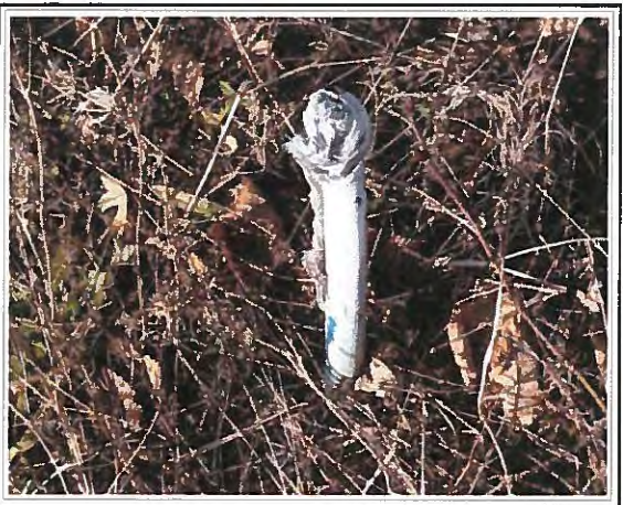
Water line for additional cabins
