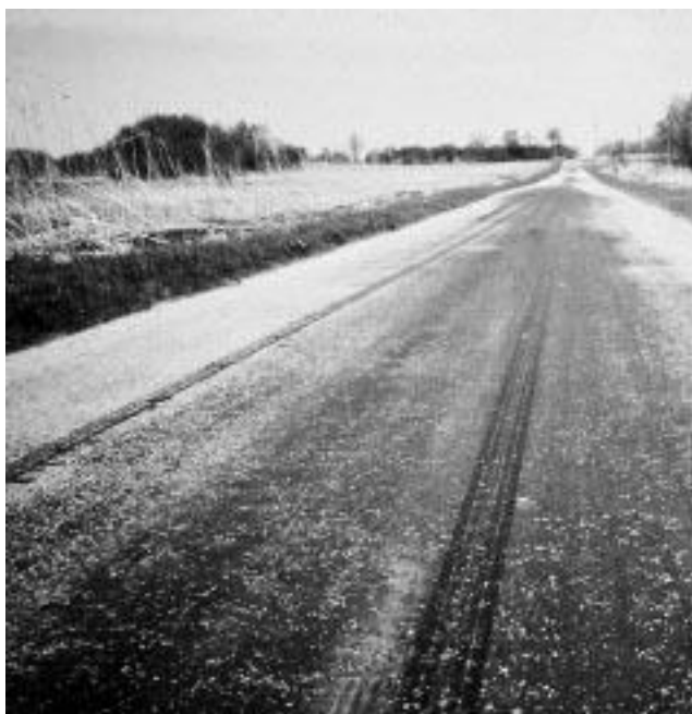
▼ Severe flushing.
