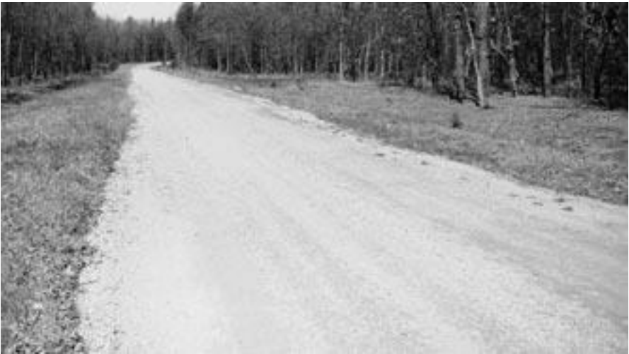
◀ Adequate gravel layer. No ruts or potholes.
