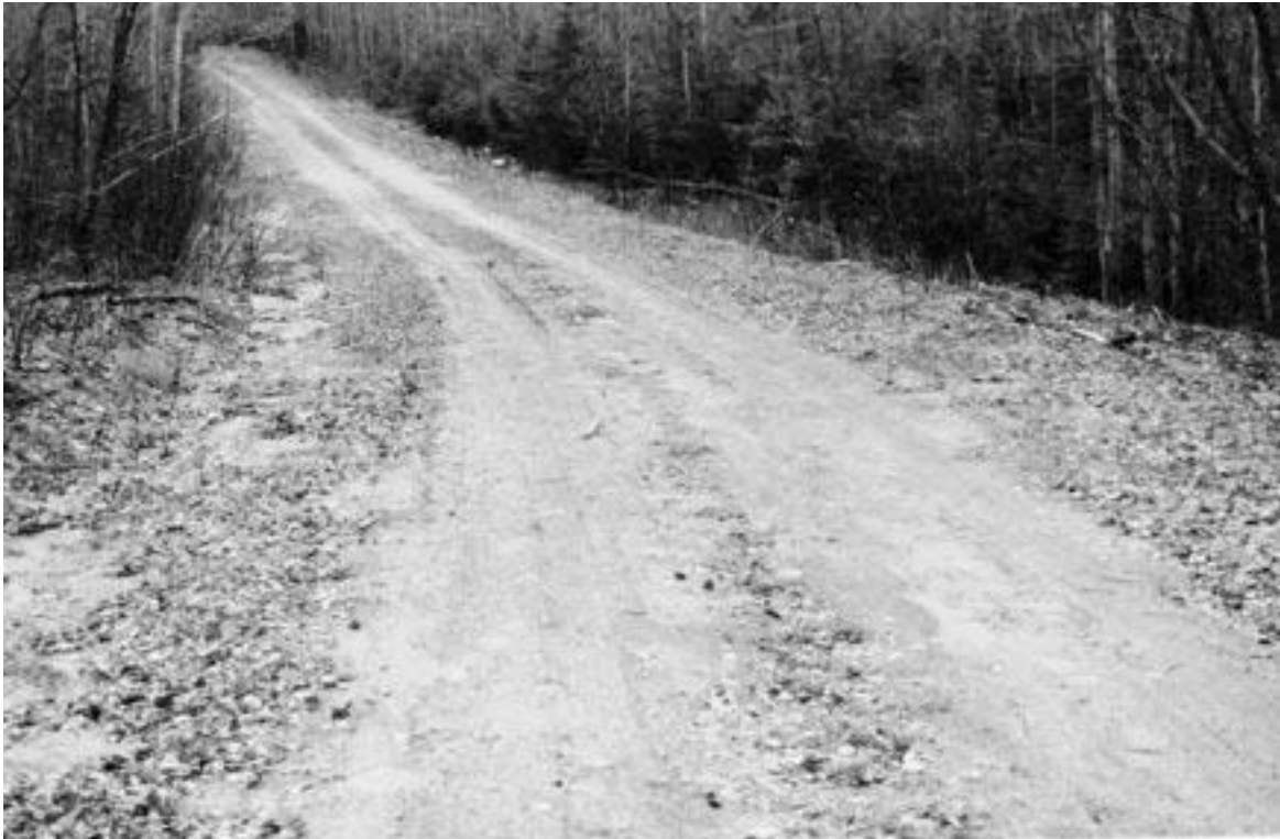
◀ Adequate gravel layer. No ruts or potholes.
