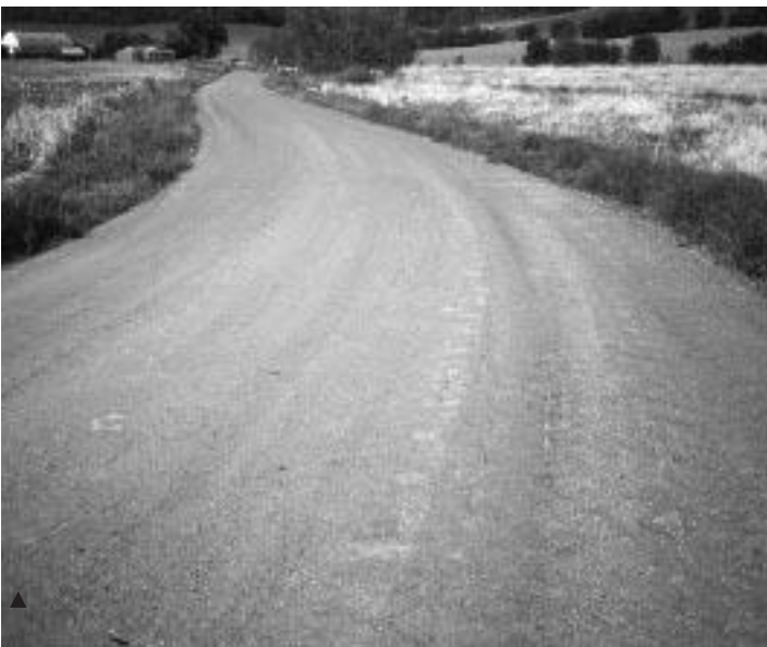
New cold mix surface.
