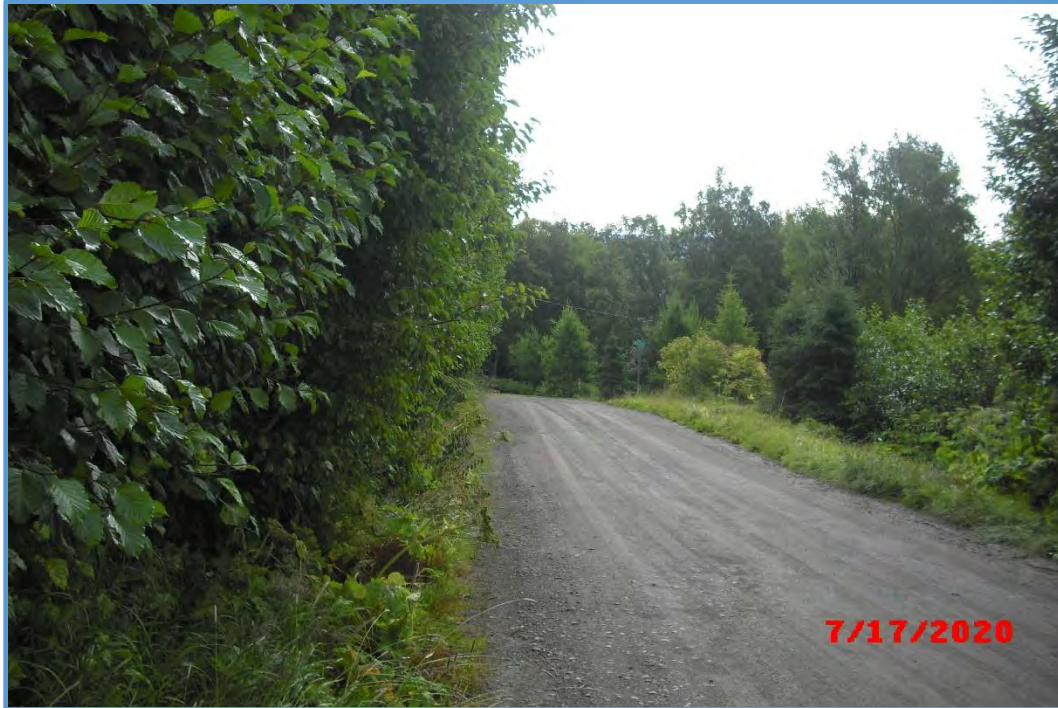
Figure 9: Alder, routinely hedged, yet impeding ditch establishment due to road misalignment
