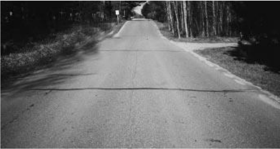
▼ Widely spaced, well-sealed cracks.
