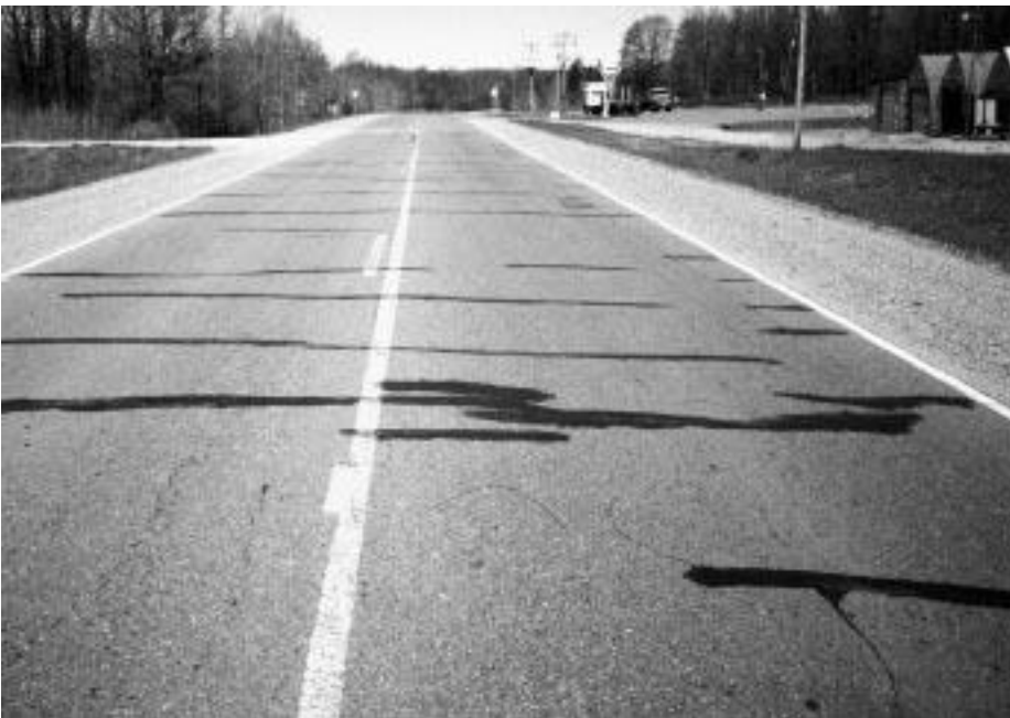
◀ Sealed cracks, a few feet apart.
