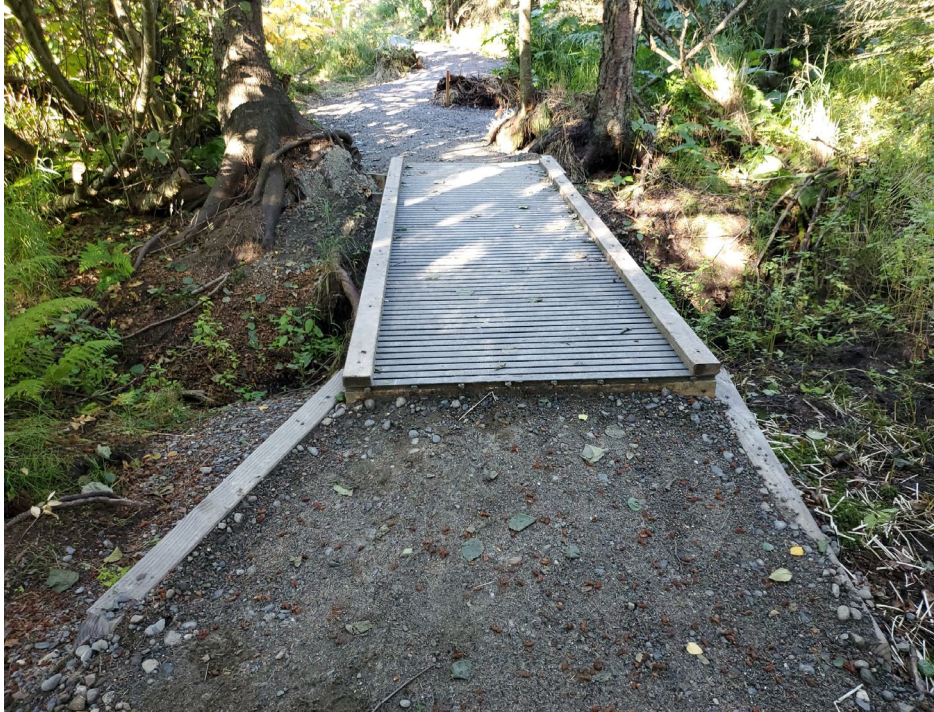
Bridge lip where a metal transition plate will be installed.
