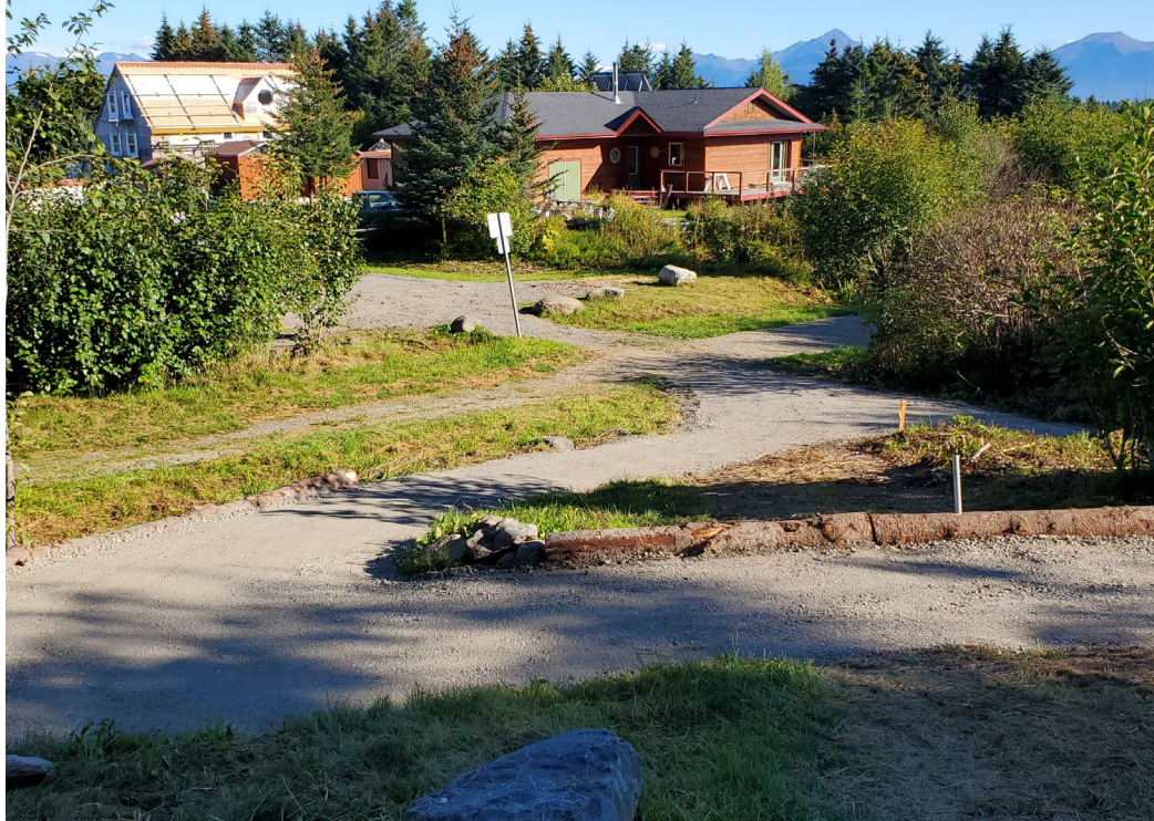
Switchback where trail was widened, grade reduced, and bumpers installed.
