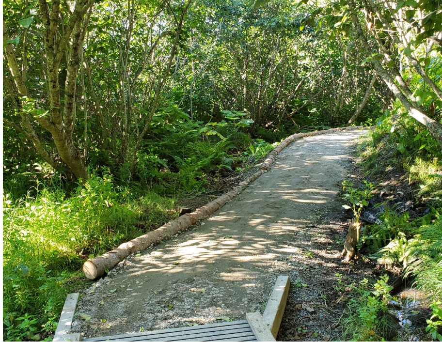
Spruce round trail bumpers installed along trail.
