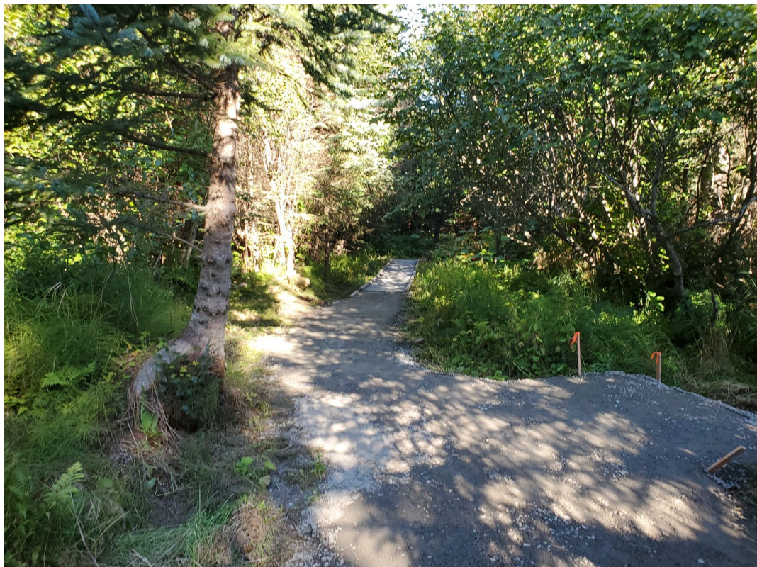
Widened area where a bench will be installed.
